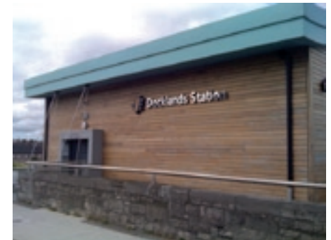
Docklands Rail Station
