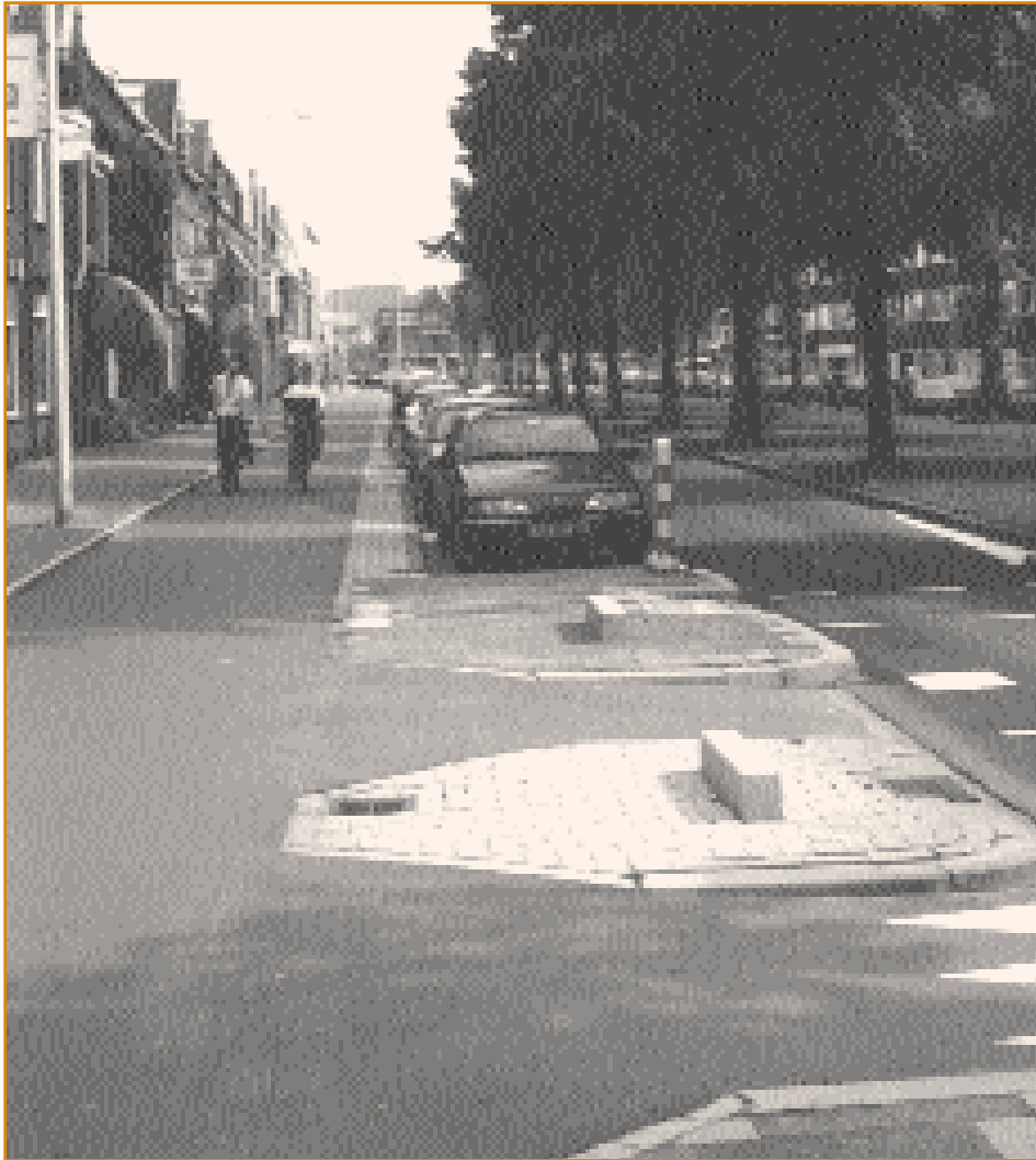
Segrated Cycle Facility and Exit Construction (Holland)
