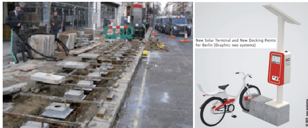
Figure 12 The disruption caused by conventional docking station implementation (left) and a potential low impact, low cost, solar-powered, concrete alternative (right)
