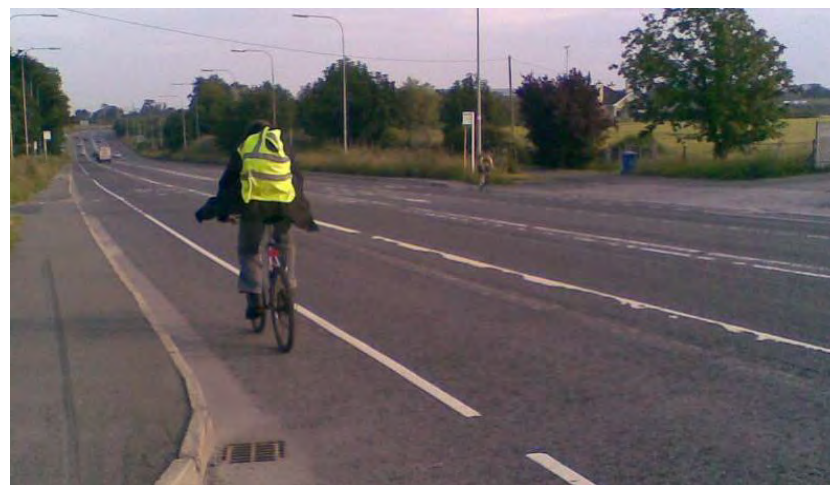
Cycle Lane on R132 Swords Road between Swords and Dublin Airport (QoS score of D due to lack of segregation from high-speed traffic and narrowness)
