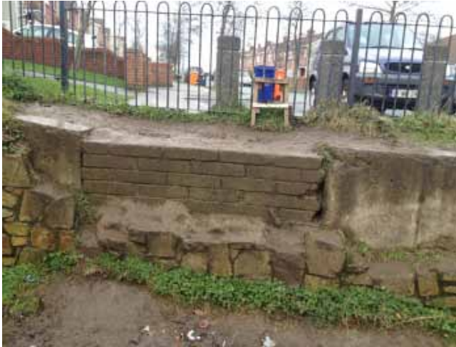
Figure 6.4: Example of damage to the public realm with creation of steps in blockwork and the construction of a 'stile' to climb the railing. This is located on a desire line from a housing estate to the local school in Rathcoole, Co. Dublin.
