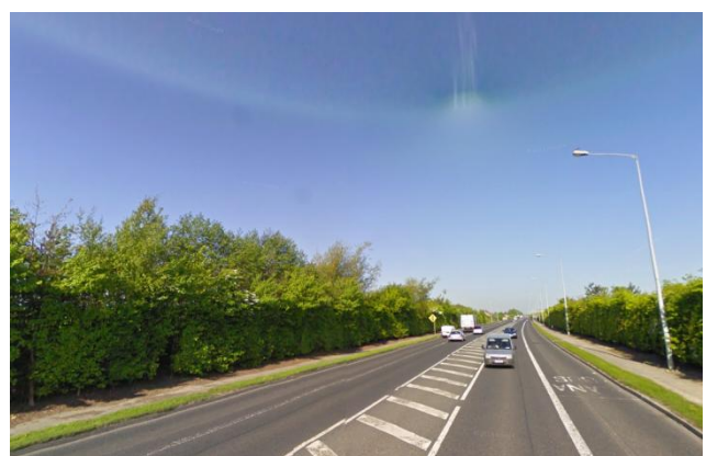
Figure 9.4 Existing, but not operational, bus lanes on the R139
