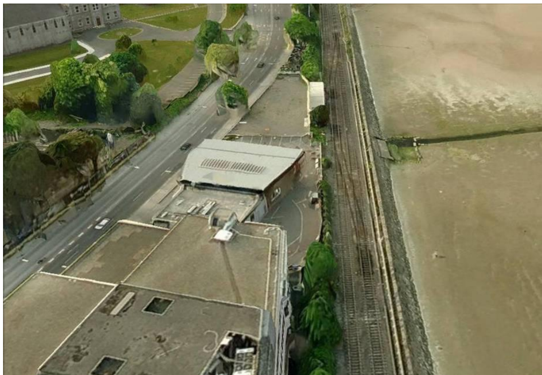
Confined Corridor on Inland Side of Railway at Merrion Petrol Station and Offices
