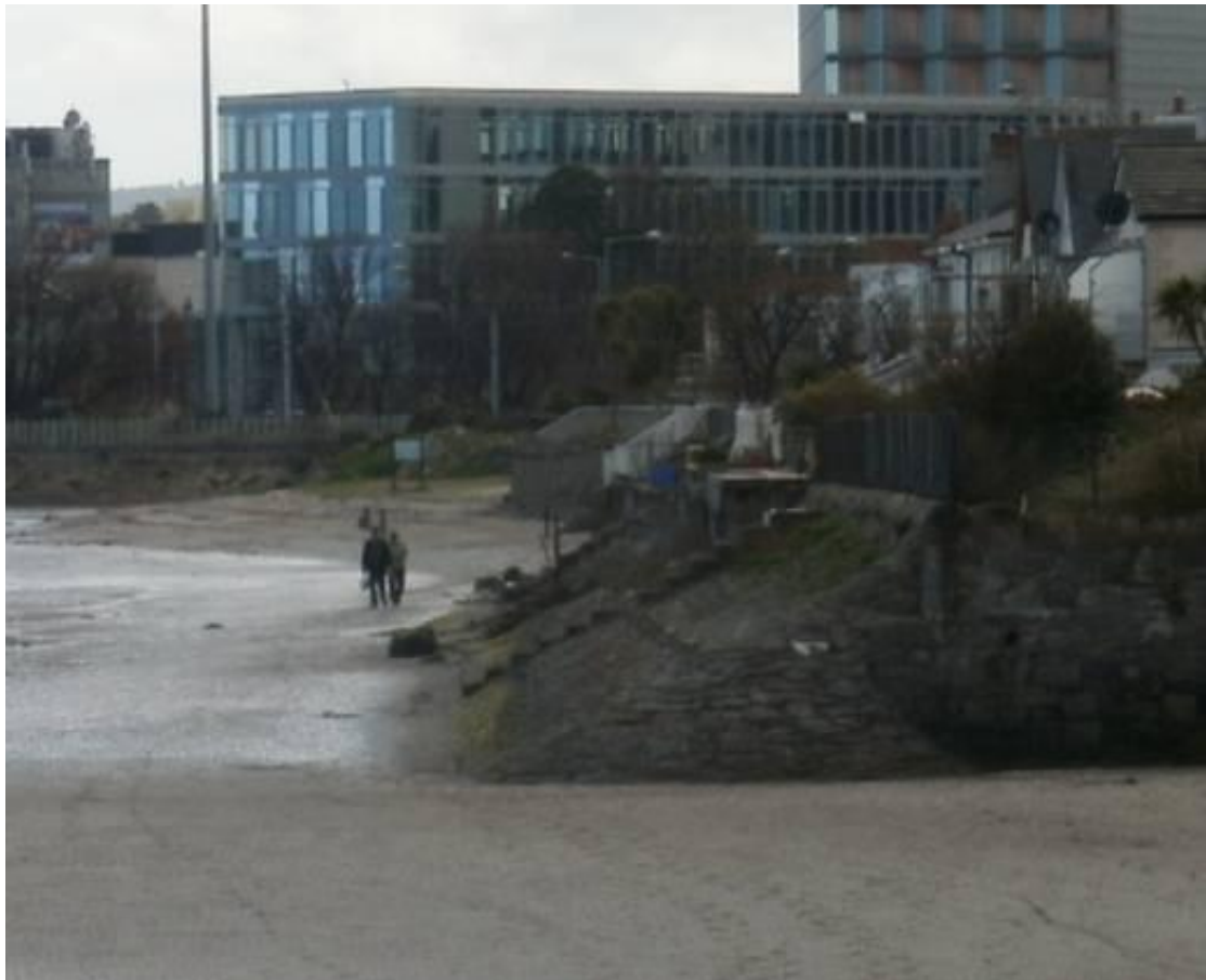
Close-up view of seaward side of houses at Merrion Strand with stone revetment
