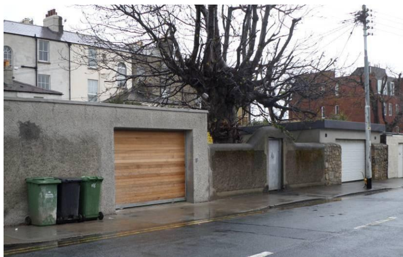
Typical Situation on Northern side of Seapoint Avenue at rear of Ardenza Terrace
