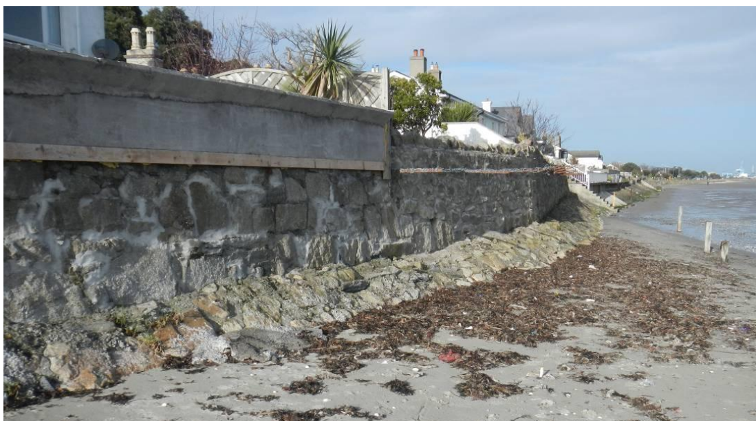
Vertical Seawall at houses at southern end of Strand Road
