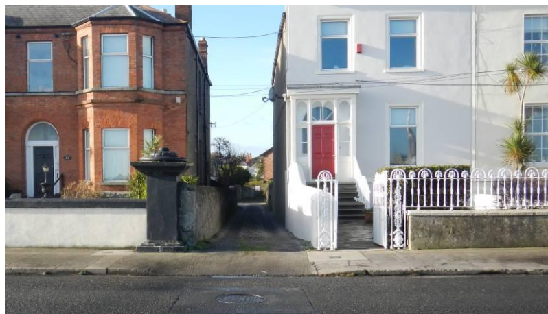
Informal Parking at houses on Strand Road - rear access available from laneway
