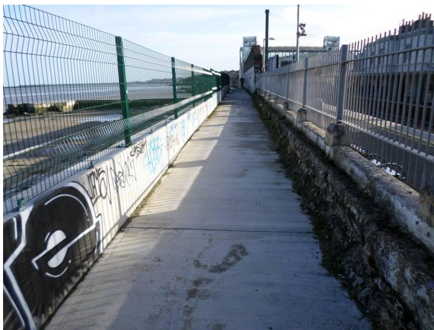
Existing coastal path at demolished Blackrock Baths
