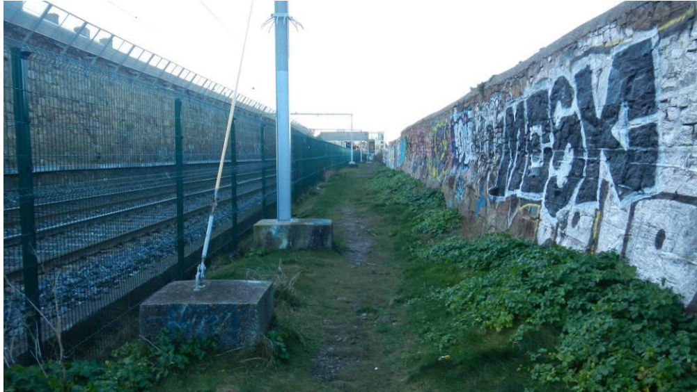
Space between Railway and Seawall East of Blackrock
