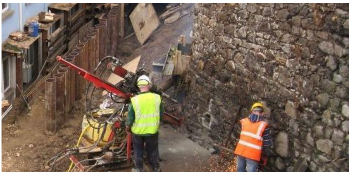
Mini-Piling Rig working in a Confined Space
