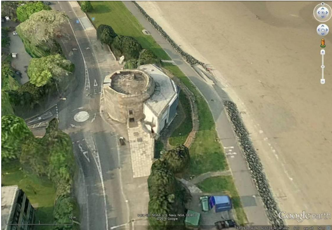
Aerial view of narrow pinch-point at Sandymount Martello Tower
