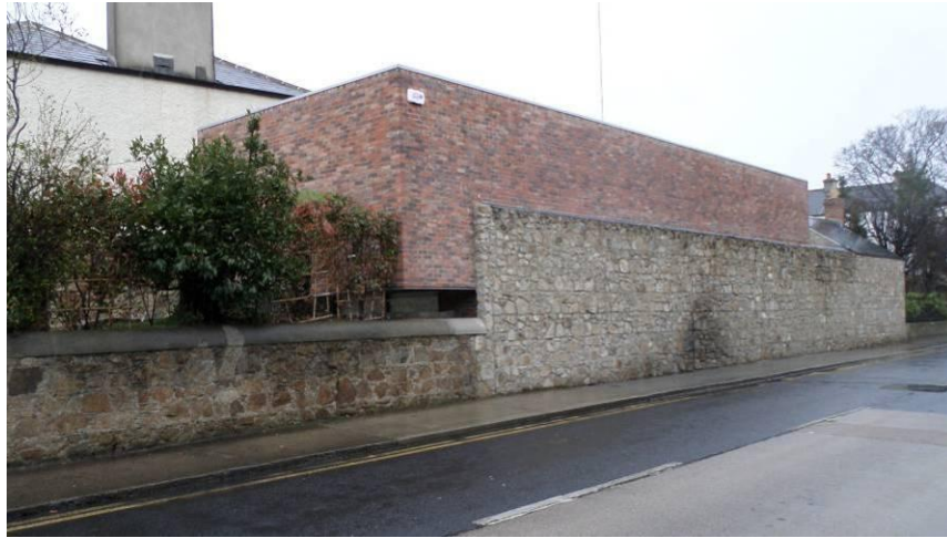
Recently constructed house on southern side of Seapoint Avenue
