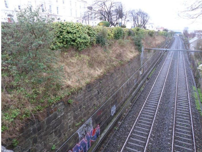
Railway Cutting at Trafalgar Terrace
