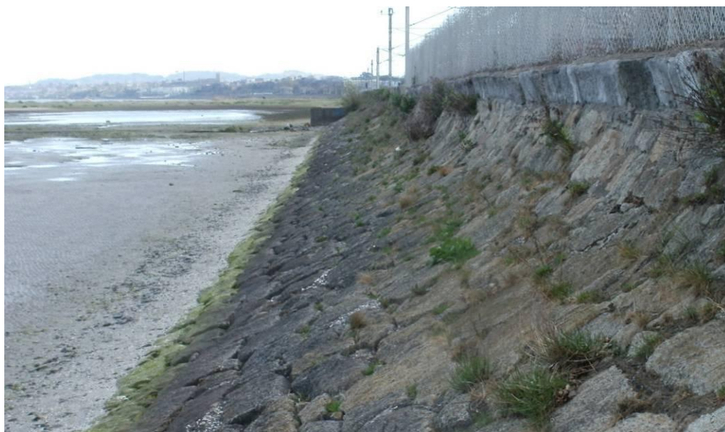
Railway Revetment north of Trimleston Sand Spit - Roughly 4m wide
