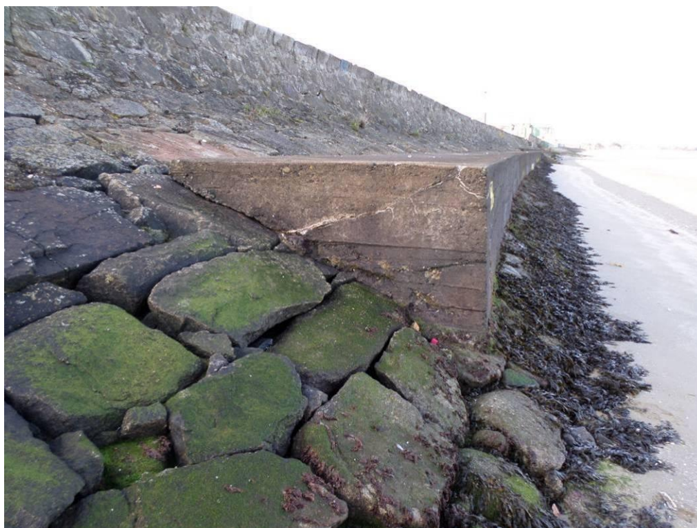
Existing 2m wide Ledge on Revetment south of Booterstown Station
