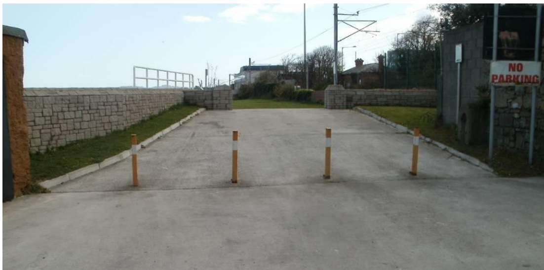
Flood Protection Ramp at Beach Access at Merrion Gates (Old Station House visible in background)
