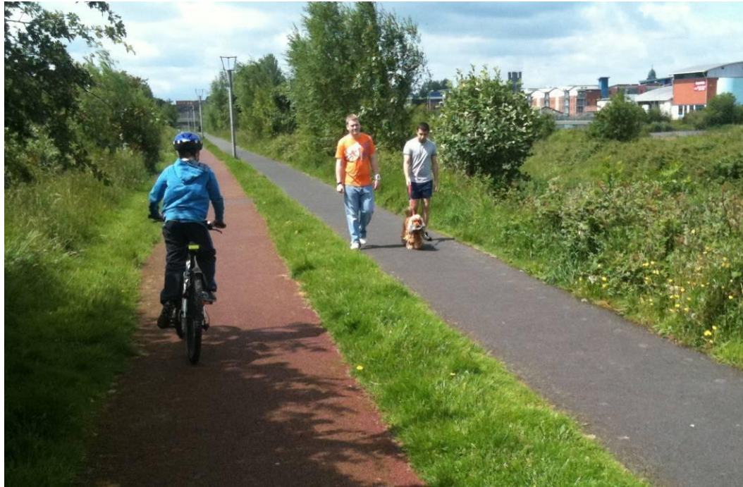
1m wide grass separator verge: Shannon Canal, Limerick
