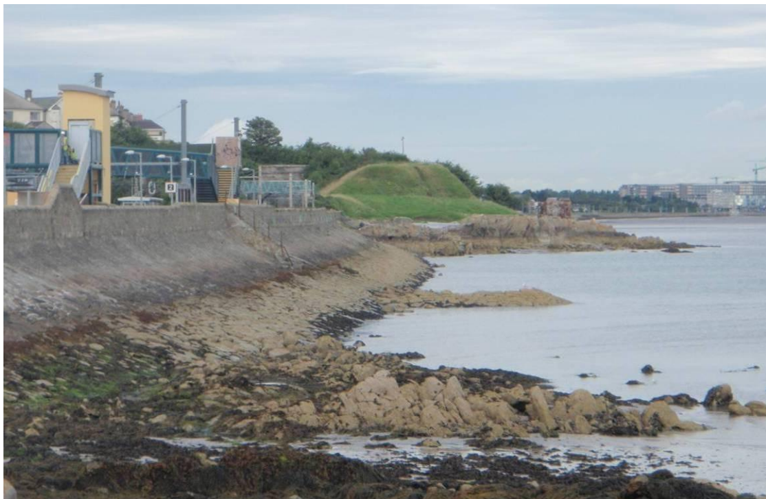
Wide Sloped Revetment at Seapoint Station
