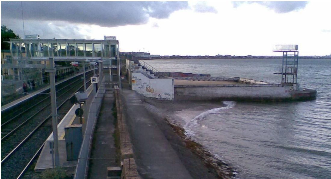
The former Blackrock Baths - now mostly demolished
