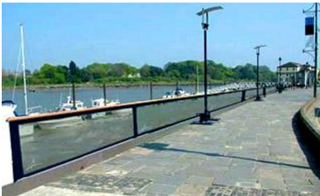
Example: Glass Flood Protection Wall in Waterford (Image from RPS)
