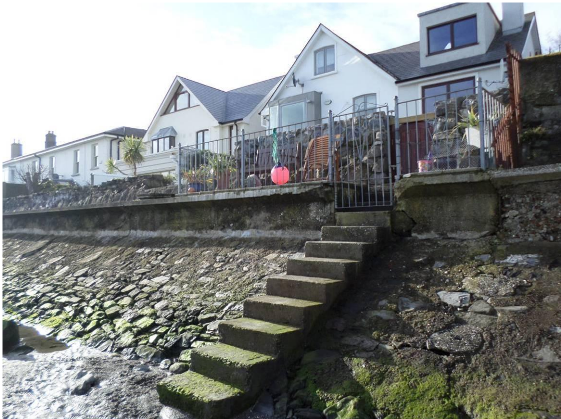
Seawall revetment at rear of houses on Strand Road midway along this section
