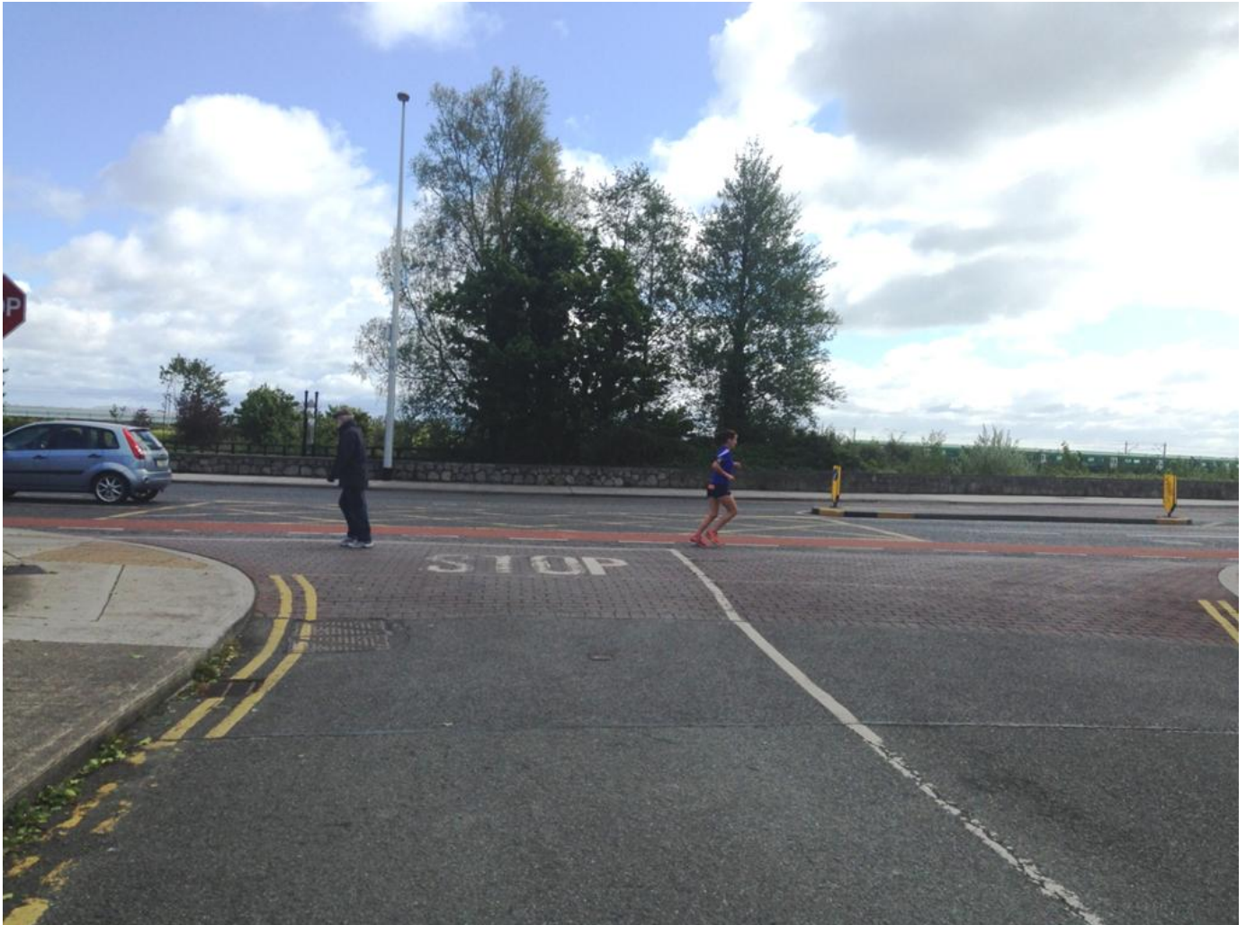
Figure 4.4 Raised crossing on St. Helens Avenue with tactile.
