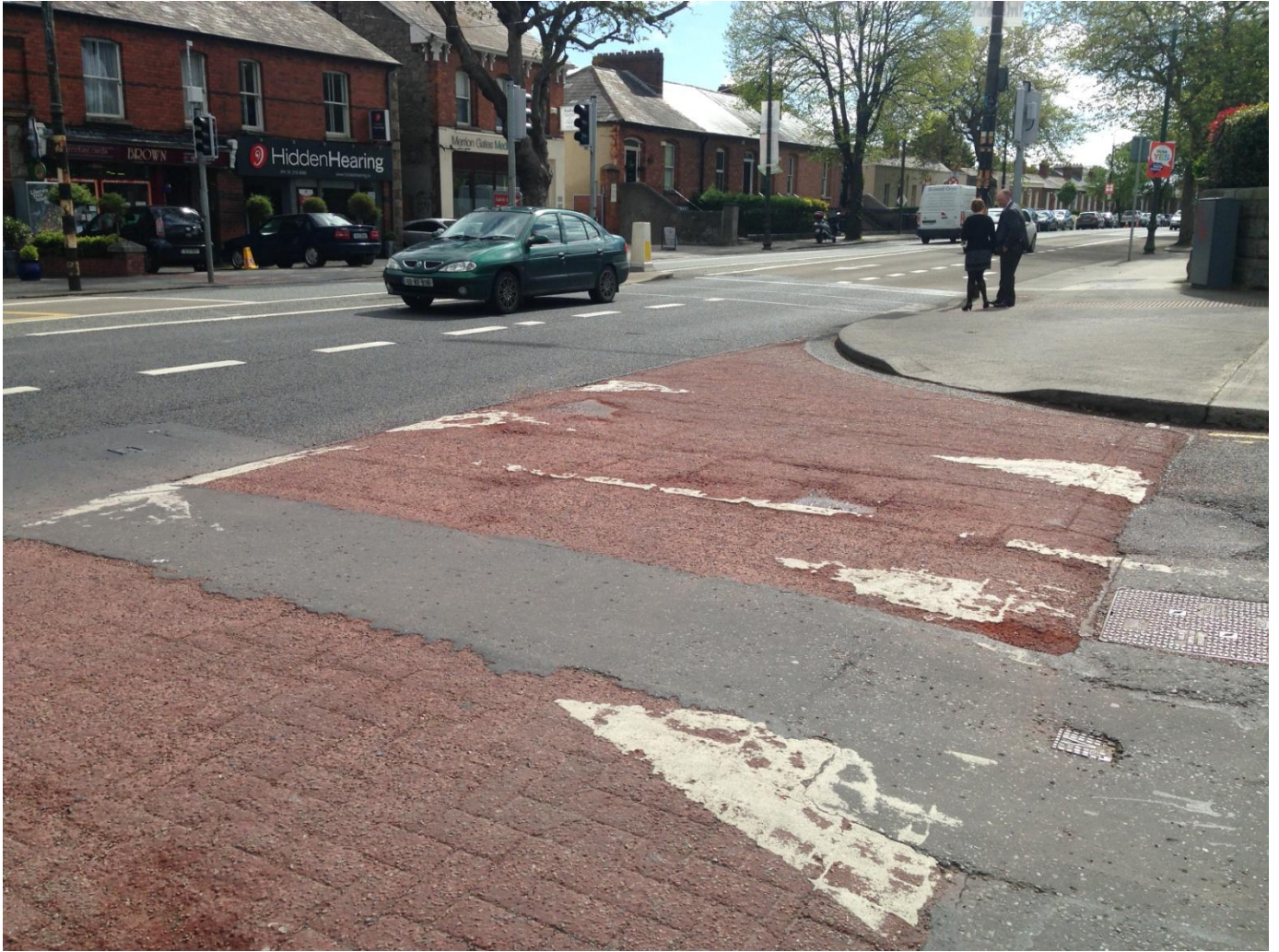
Figure 4.3 Raised Crossing on Herbert Avenue, bad state of repair, no tactile paving.
