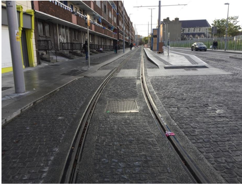
Dominick Street Lower, facing north
