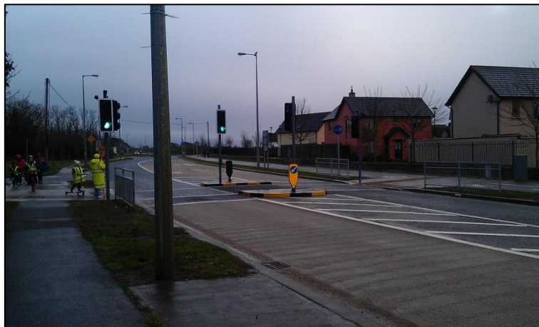
Upgraded Signalised Pedestrian Crossing
