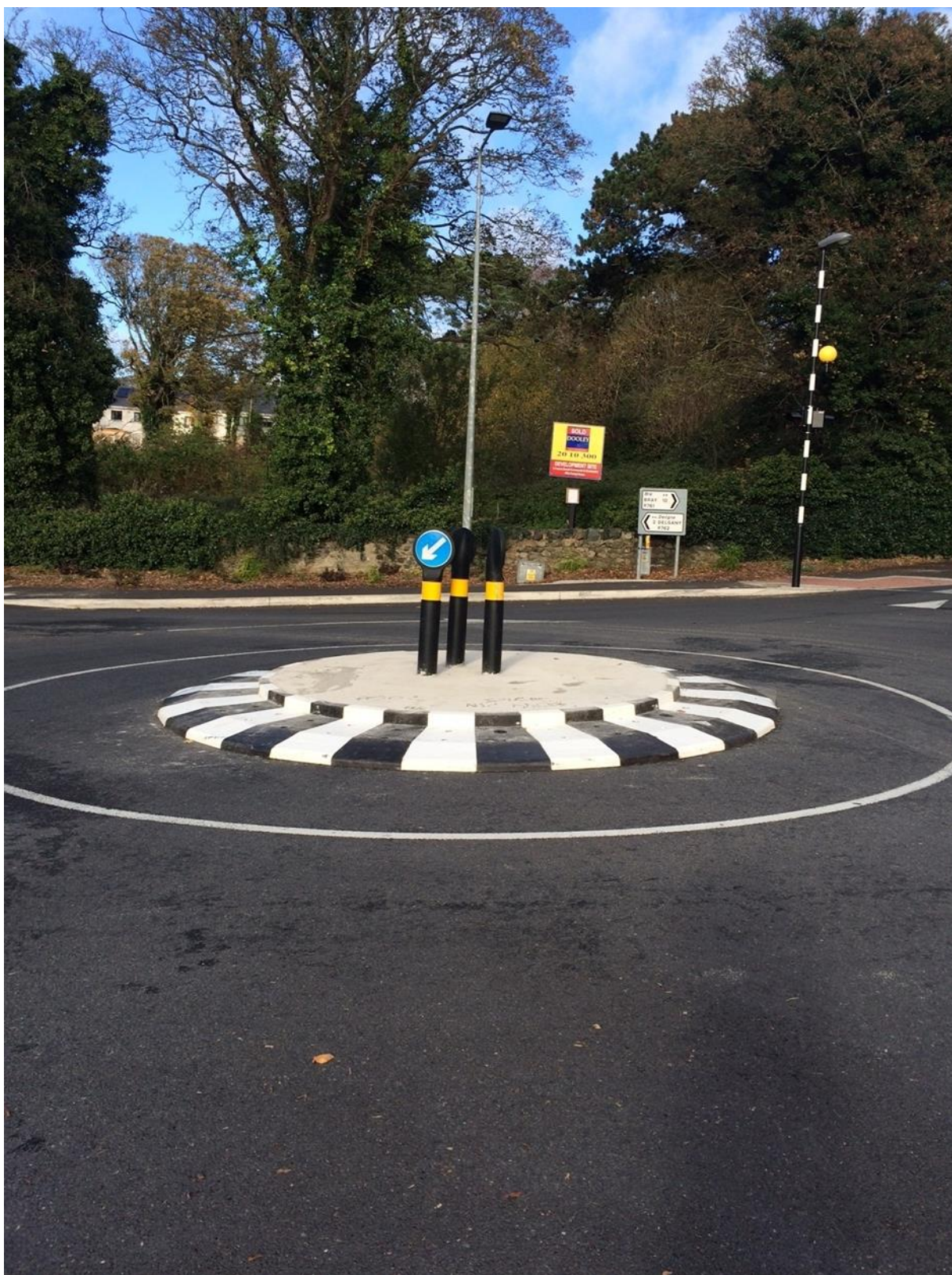
New full construction centre island with modular over-run area (northern roundabout)
