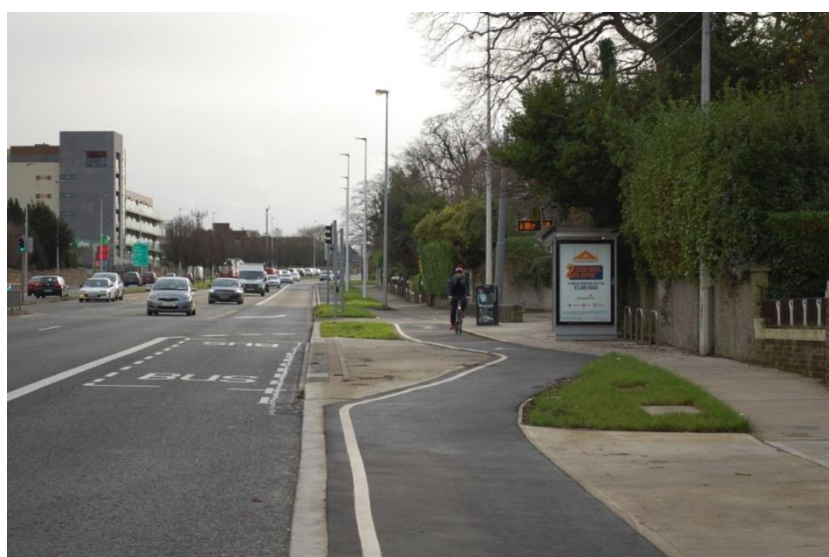
Inline bus stop with continuous cycle track and passenger set-down area
