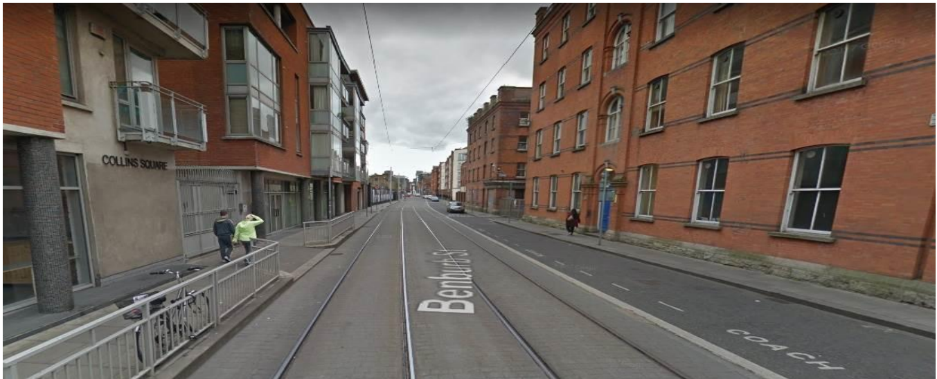
Photo 8.3 Benburb Street 1C(ii): One-way cycle track on the buildings side north of the river
