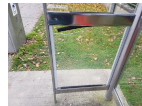
Shelter no 607801 @ University Hospital , Limerick in towards the city. Window glass broken on left hand side of shelter as you look at the shelter.
