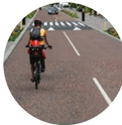
Hot rolled asphalt with red chippings
