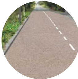
Cold applied high friction buff surface
