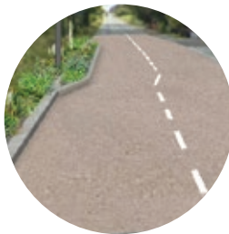
Cold applied high friction buff surface
