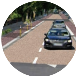
Cold applied high friction buff surface
