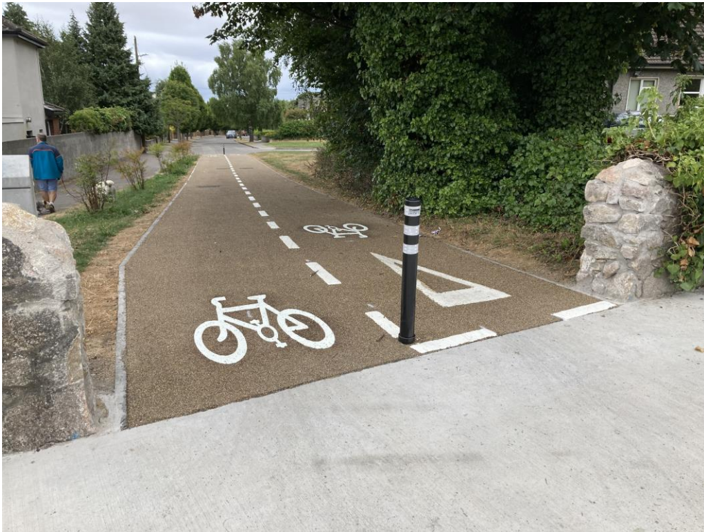
Figure 10: Wide gap with 70mm diameter bollard in the centre, with 1.5m clear space each side.
