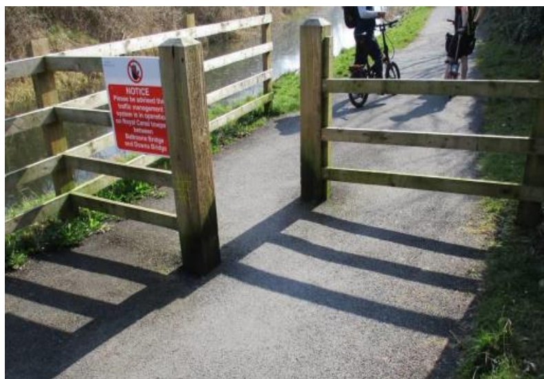
Figure 3: Staggered barriers closely space and forming a restrictive chicane
