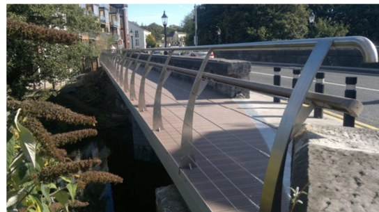
New cantilevered footpaths.
