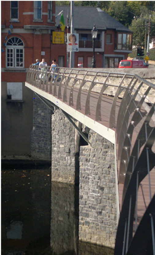
New cantilevered footpaths.
