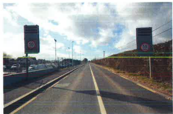
Allenwood Road (after)
