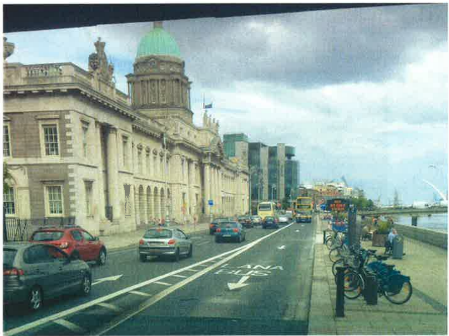
Custom House Quay contra flow bus lane
