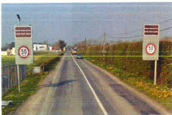
Allenwood Road (before)
