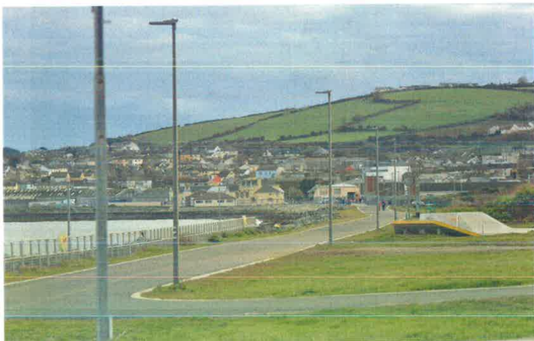
New cycle route, looking south
