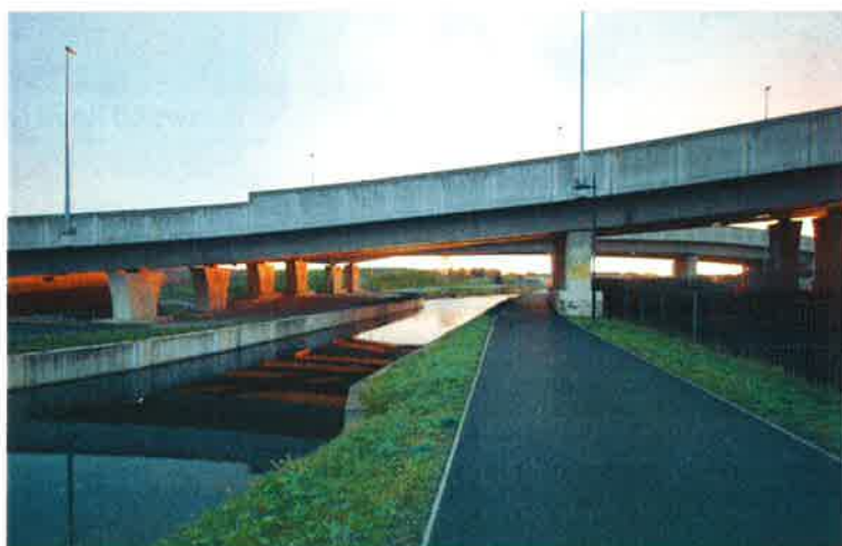
Canal towpath, facing east, showing N3-M50 junction overhead.
