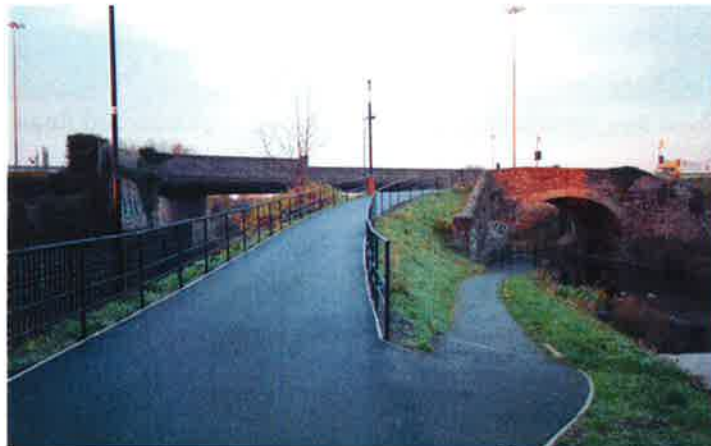
Canal towpath, facing west, showing 18 th century bridge.
