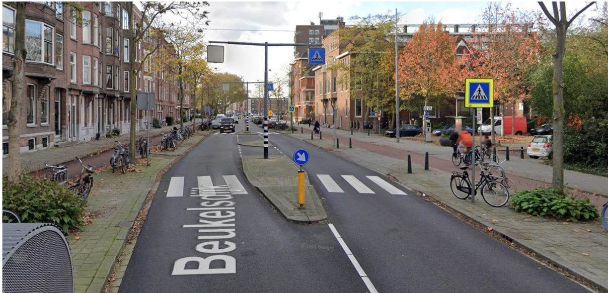
Figure 3.2: Pedestrian crossing with additional signs to increase visibility, Rotterdam (Image: Google Street View)
