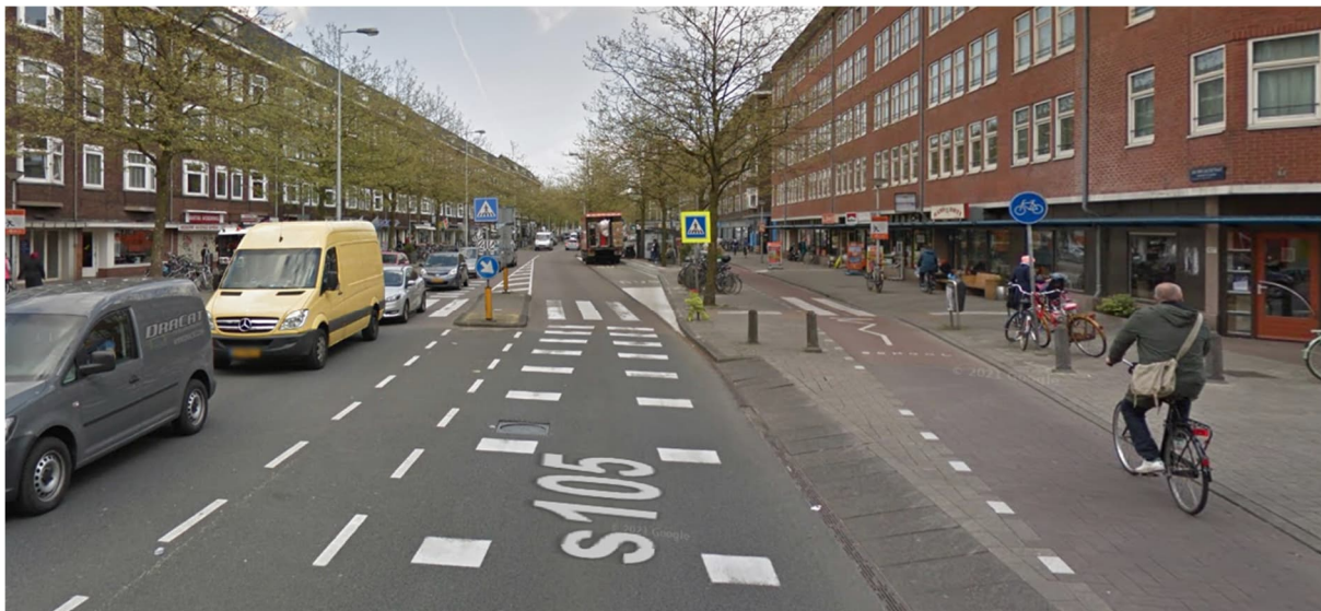
Figure 3.3: Converging road markings on approach to crossing, Amsterdam (Image: Google Street View)
