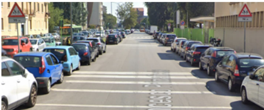
Figure 3.13: Road markings on approach to pedestrian crossing at a school zone (Image: Google Street View)
