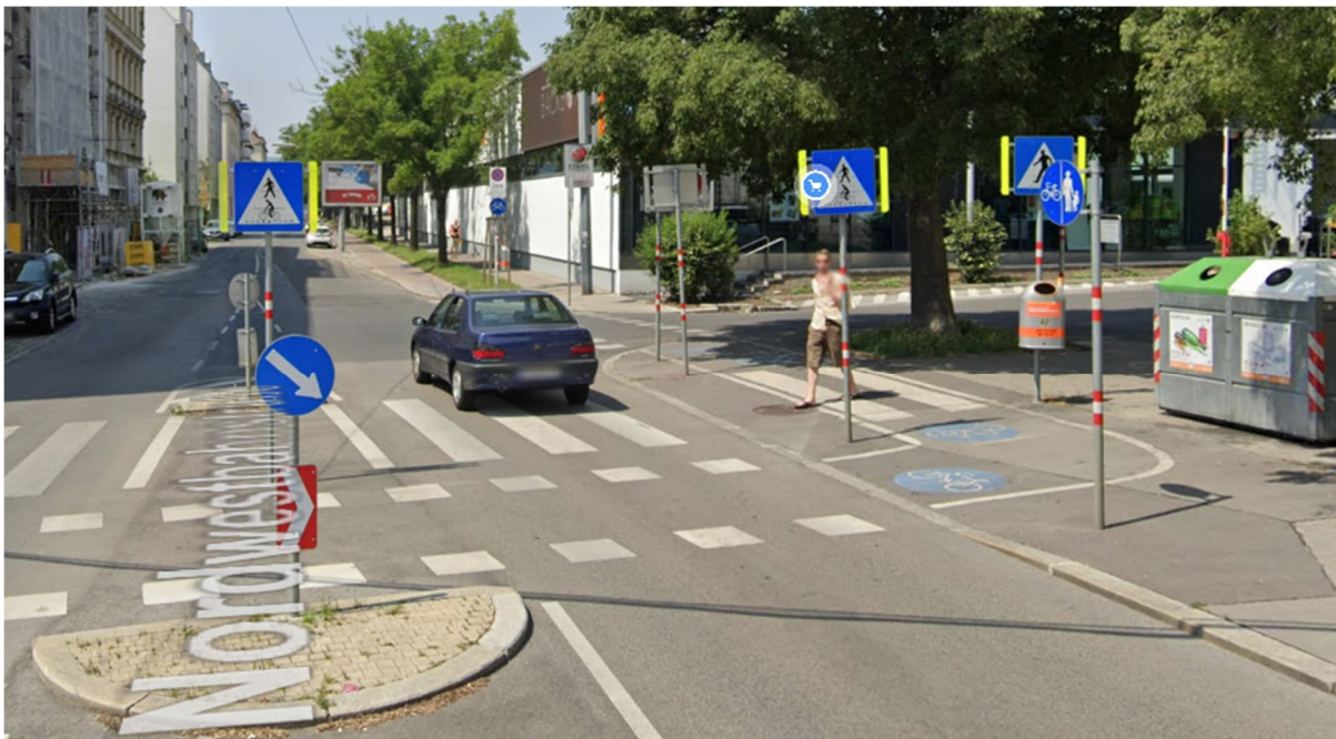
Figure 3.10: Parallel cycle and pedestrian crossing layout, Vienna (Image: Google Street View)
