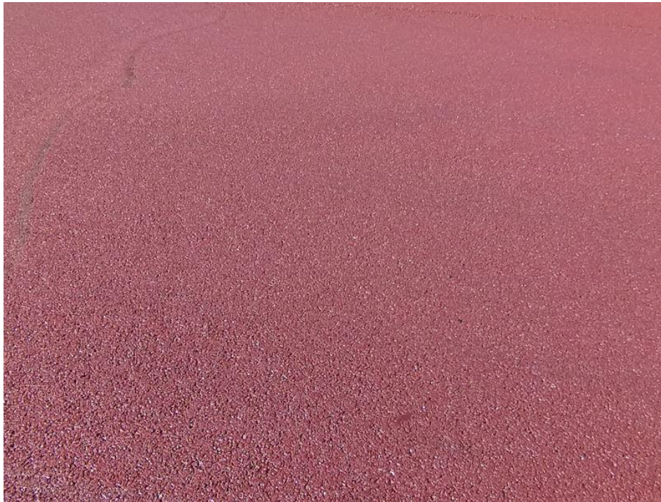
Figure 2: Stone Mastic Asphalt for Urban Cycleways – Example of Typical Red Colour (RAL 3013) to be Achieved
