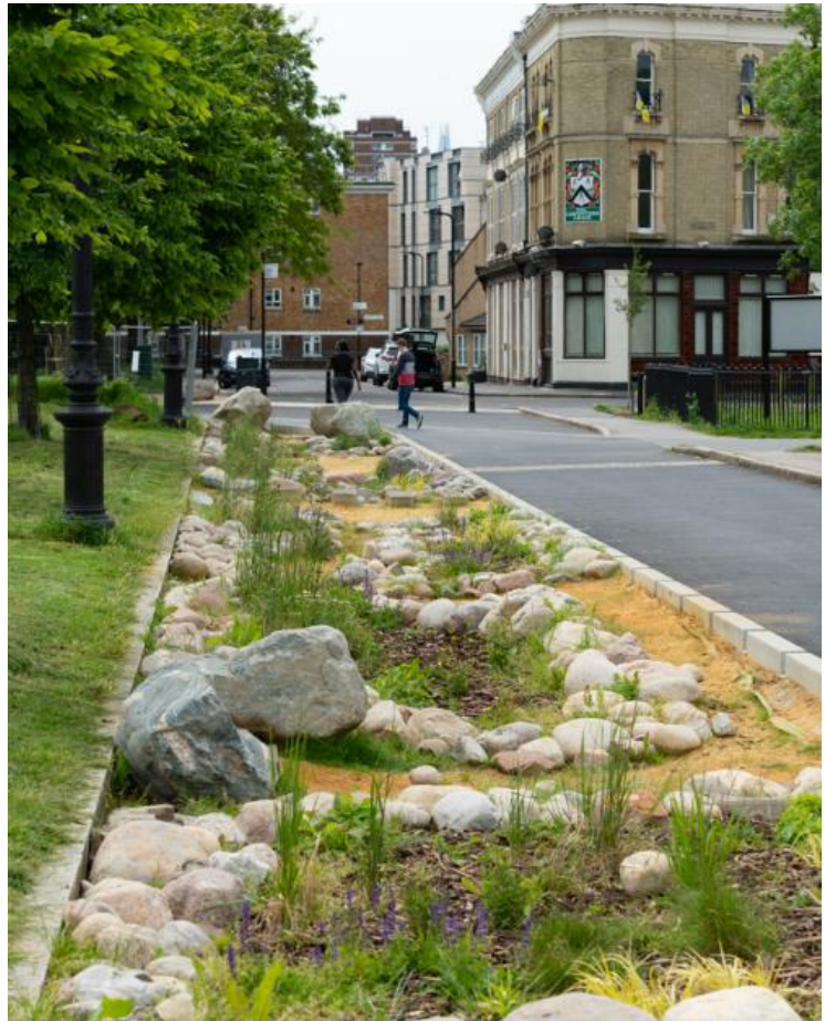
Figure 1 Typical example of recently constructed SuDS features in the form of rain gardens Shoreditch Park, London UK
