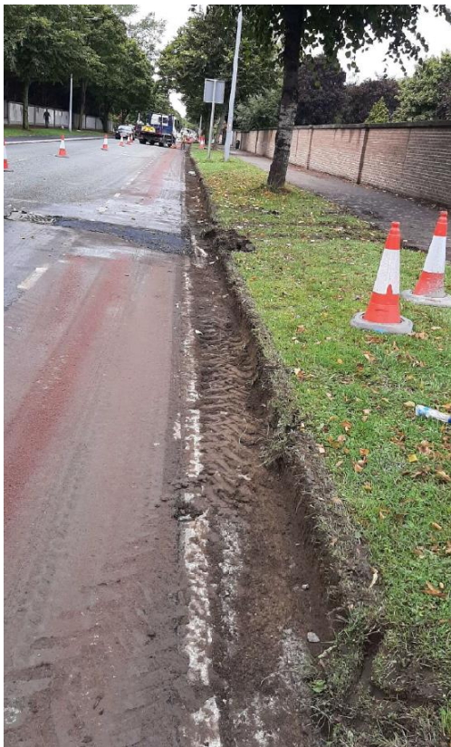
Figure 7 Original kerb milled and removed off site.
