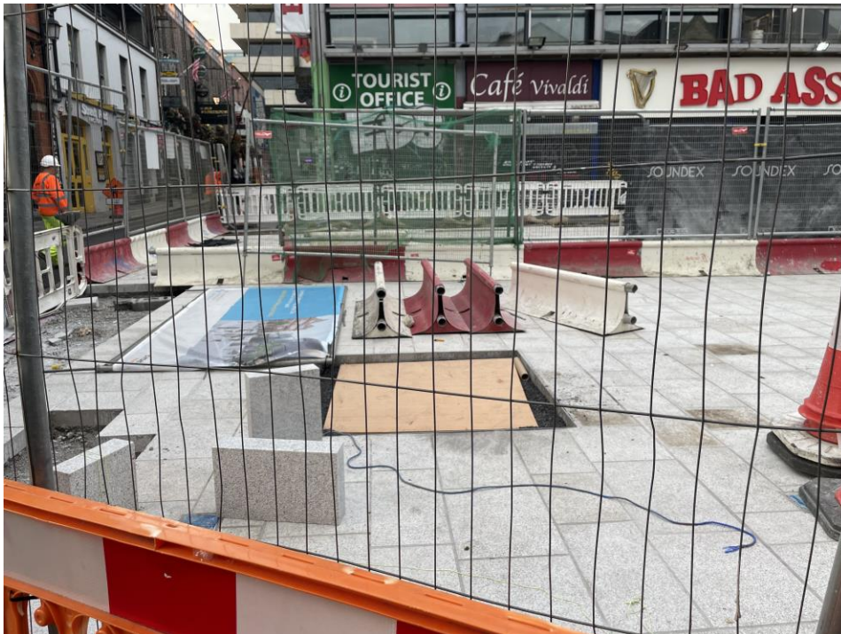
Figure 28 Temple Bar Square improvement scheme - crate system Work In Progress
