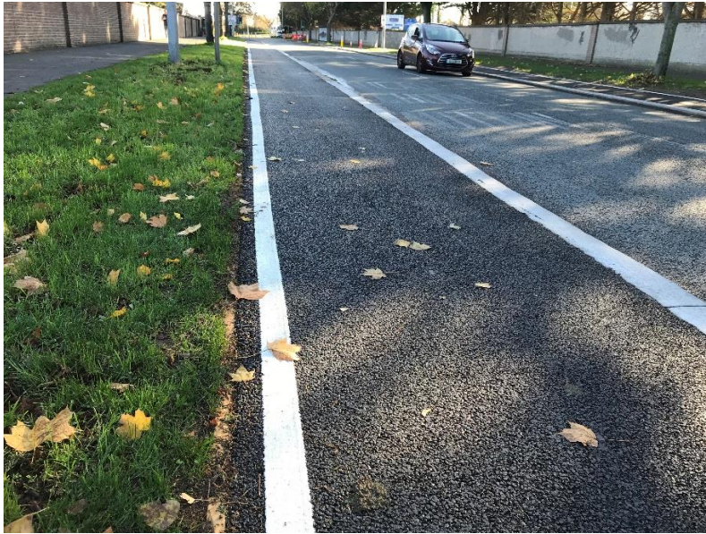
Figure 6 Image of recently implemented works at Templeville Road (R112), South Dublin
