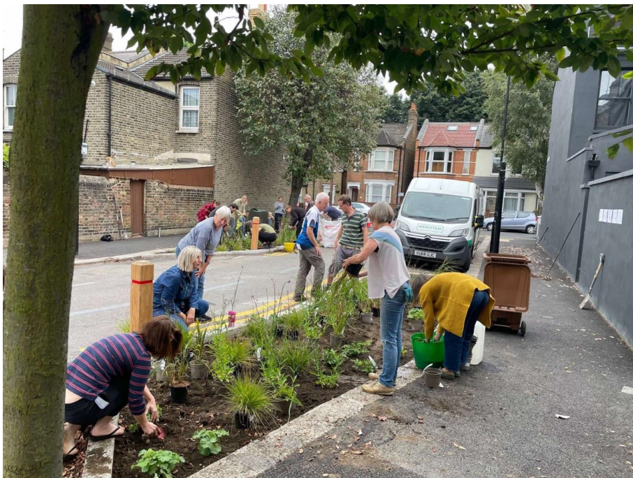
Figure 36 Community Rain Gardens project in Waltham Forest, UK - image © Meristem Design
