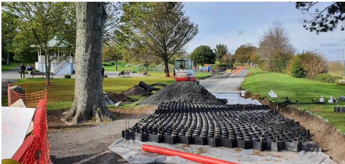
Figure 10 Shared path under construction using a no-dig solution, Blackrock Park, Dublin.
