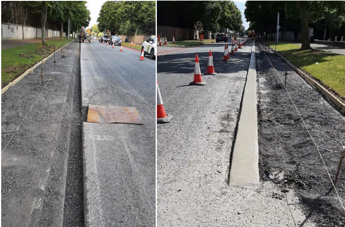
Figure 8 Construction and installation stage of the new curb maintaining greening.
