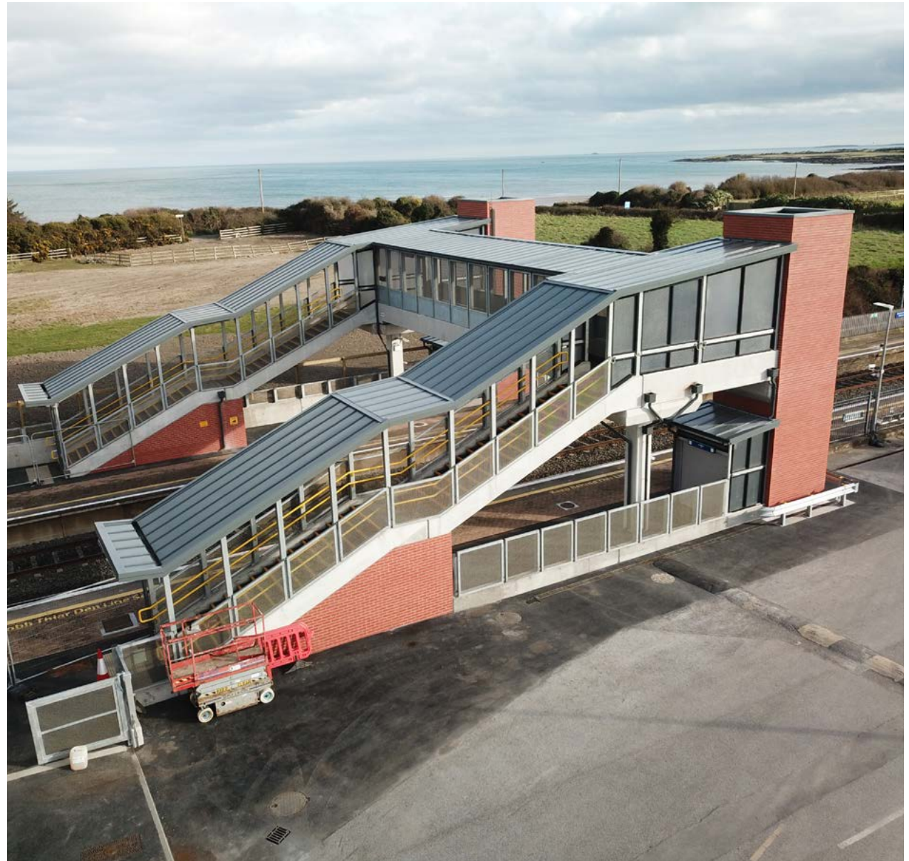
Gormanstown Lifts and Bridge
