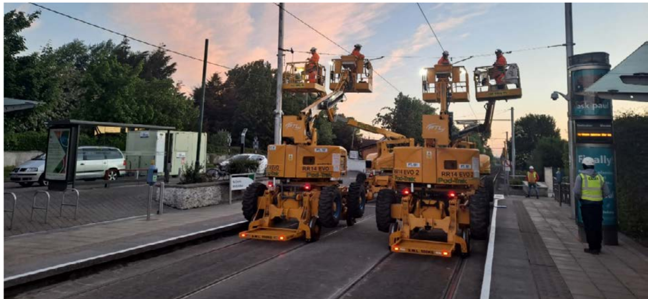
Overhead line replacements - Stillorgan
