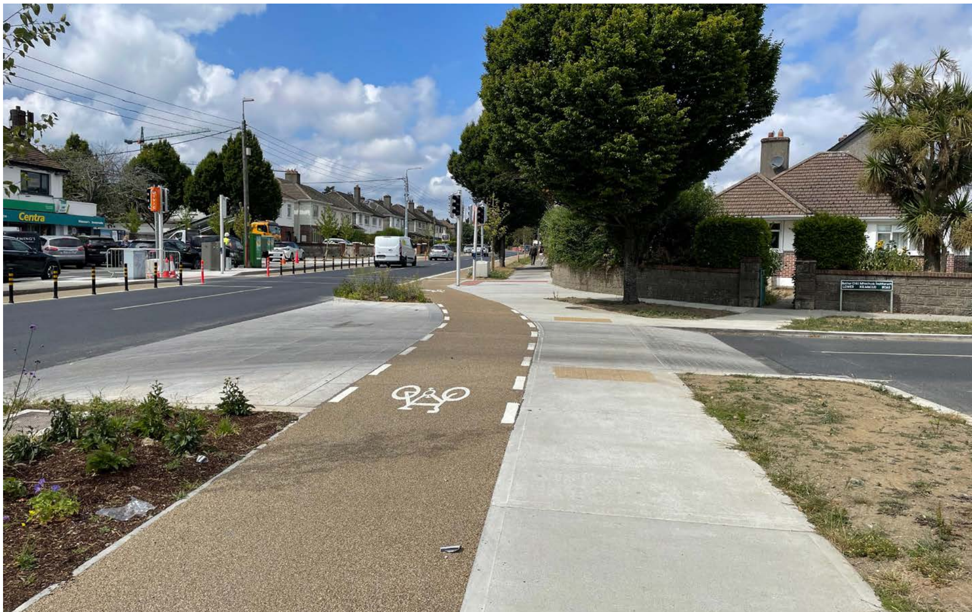
Continuous footway across a junction on Lower Kilmacud Road
