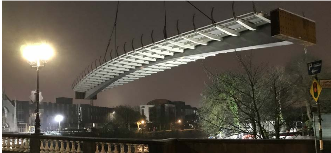
Main Span being swung into place - December 2022
