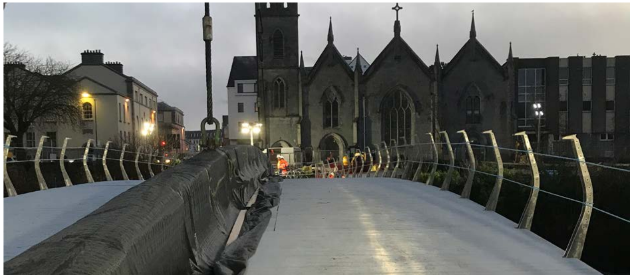
Salmon Weir Bridge, Galway
