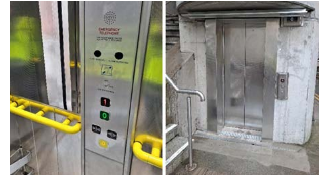
Passenger Lift Upgrade - Charlemont
