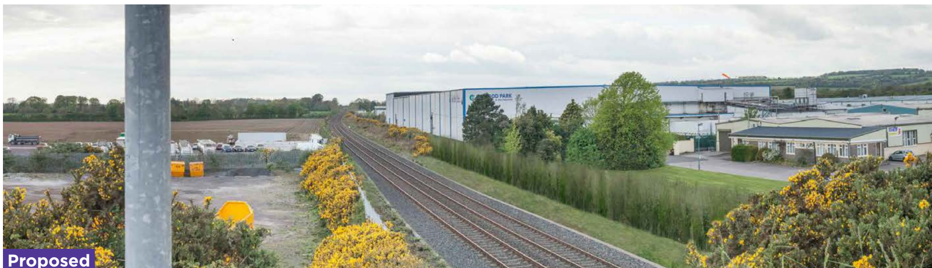
Glounthaune to Middleton Line, Middleton Northern Relied Road, Knockgriffin.
