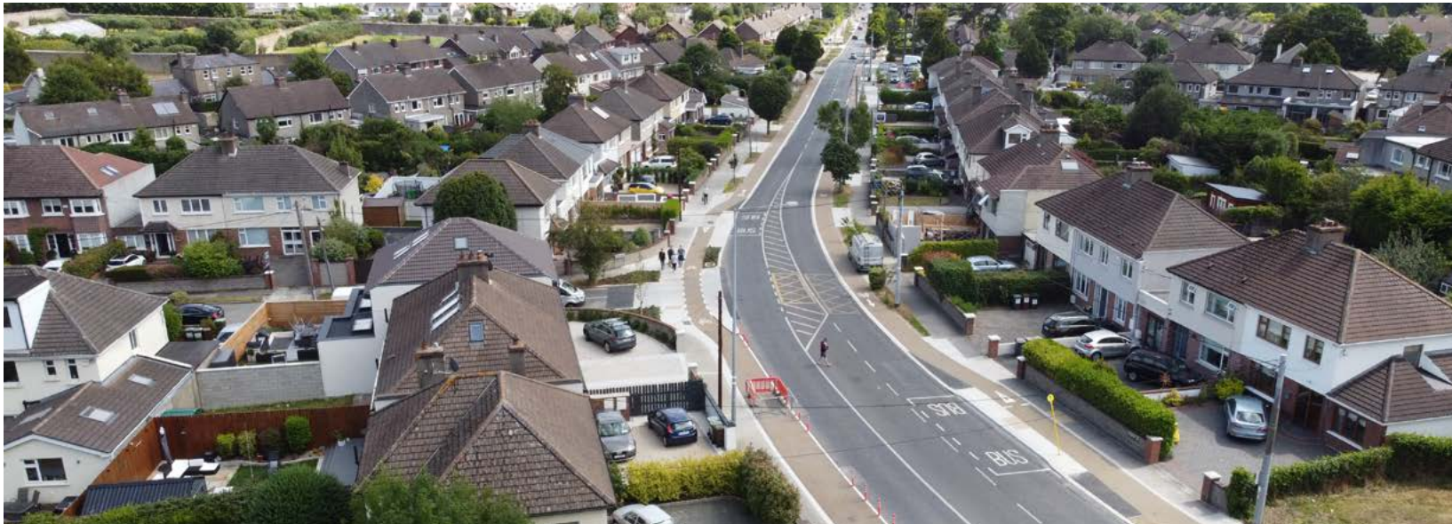
Lower Kilmacud Road
