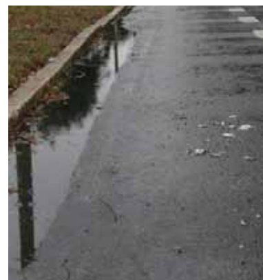
Poor drainage maintenance
