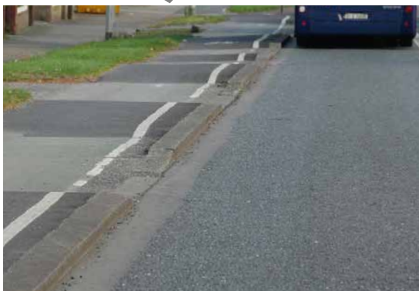
Uncomfortable and potentially dangerous surface due to driveway apron
