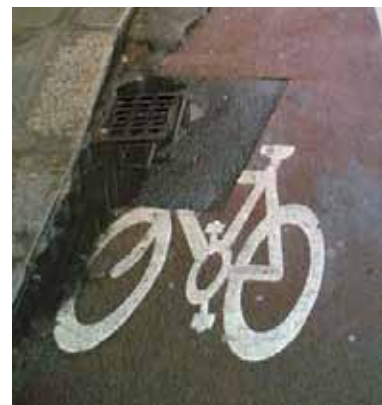
Substandard reconstruction
