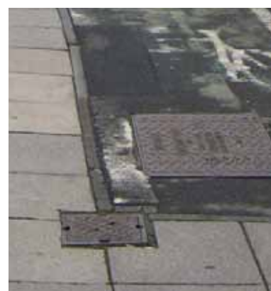
Poorly located ironmongery
