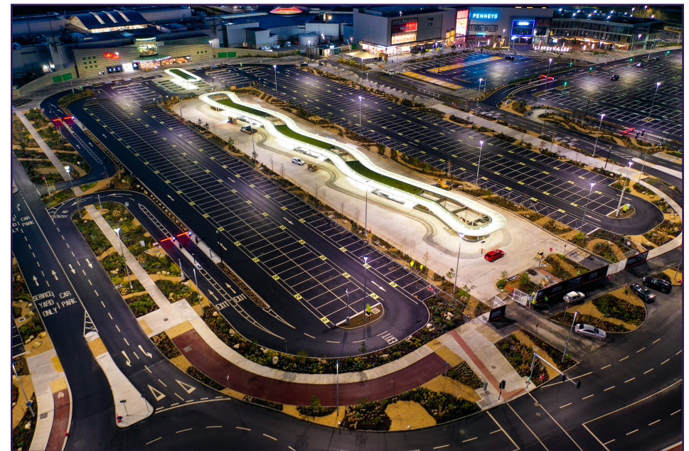
In Dublin's Liffey Valley, a spacious bus hub was built as part of a car park and shopping centre redevelopment.
