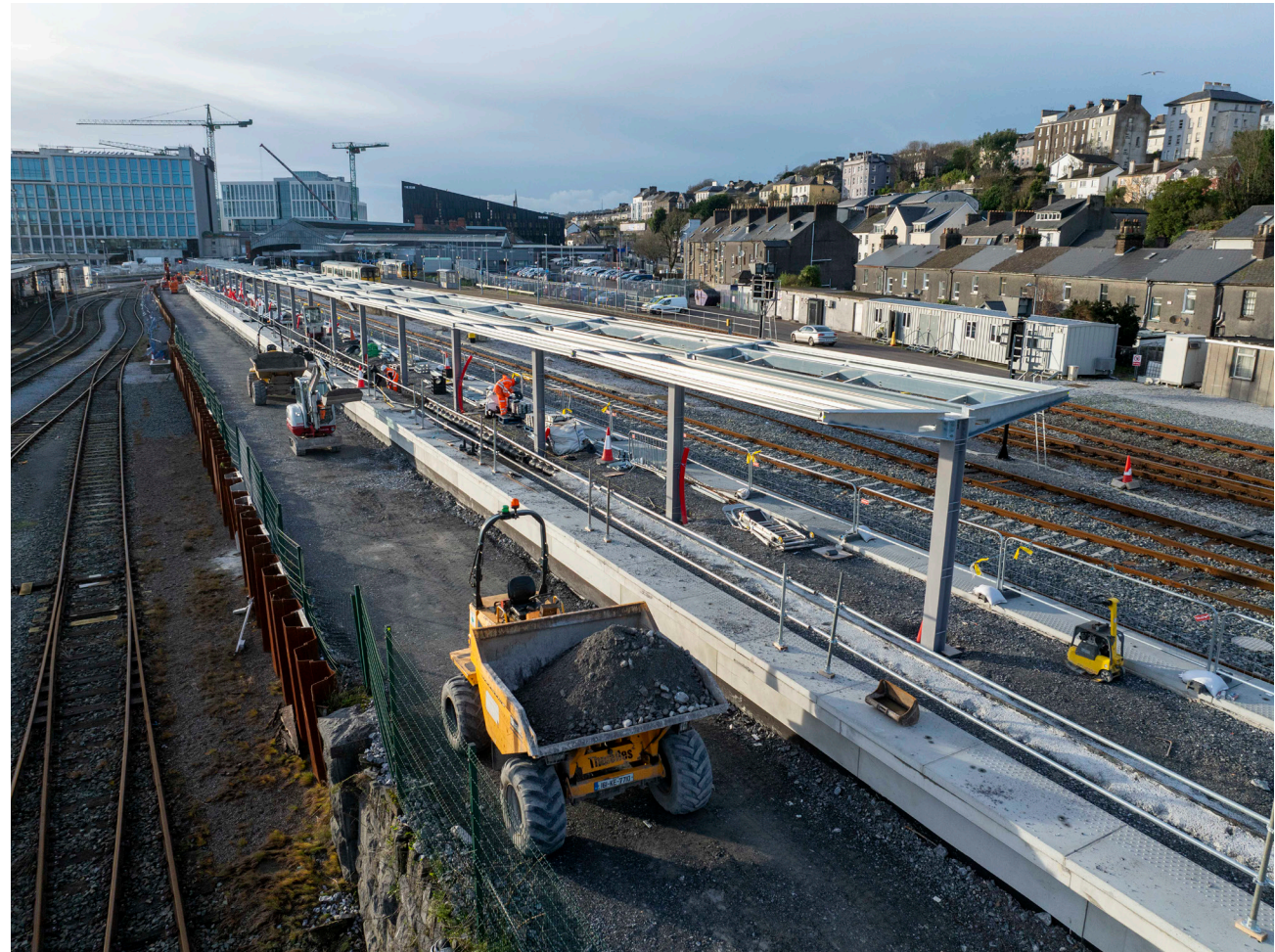
Cork Kent Station - Additional Platform Construction Work Works
