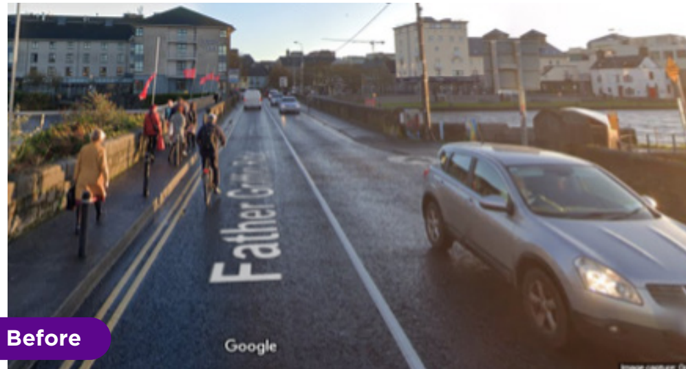
Existing Wolfe Tone Bridge
