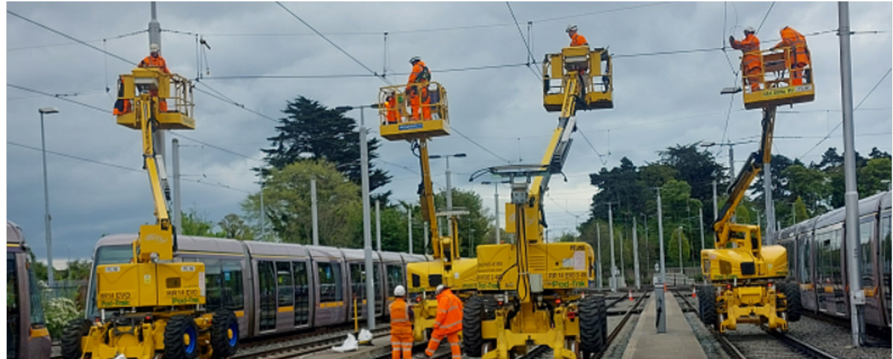
Overhead line replacement
