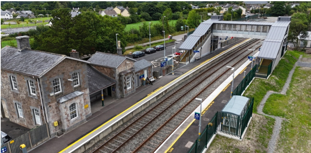
Rail Accessibility Lift and Bridge Banteer
