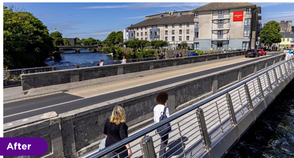
Wolfe Tone Bridge with the new cantilever section
