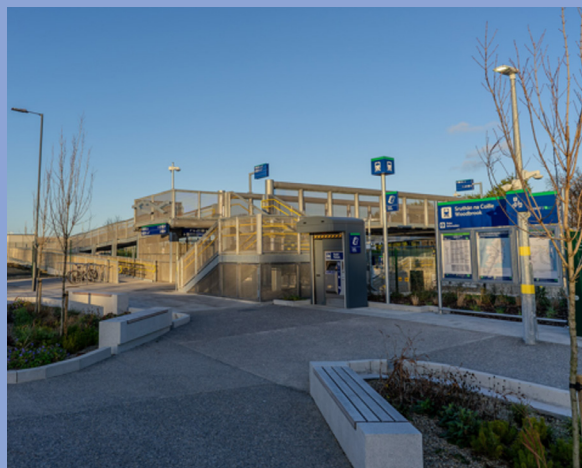
Opening of Woodbrook DART Station Woodbrook Dart Station Opened in August 2025
