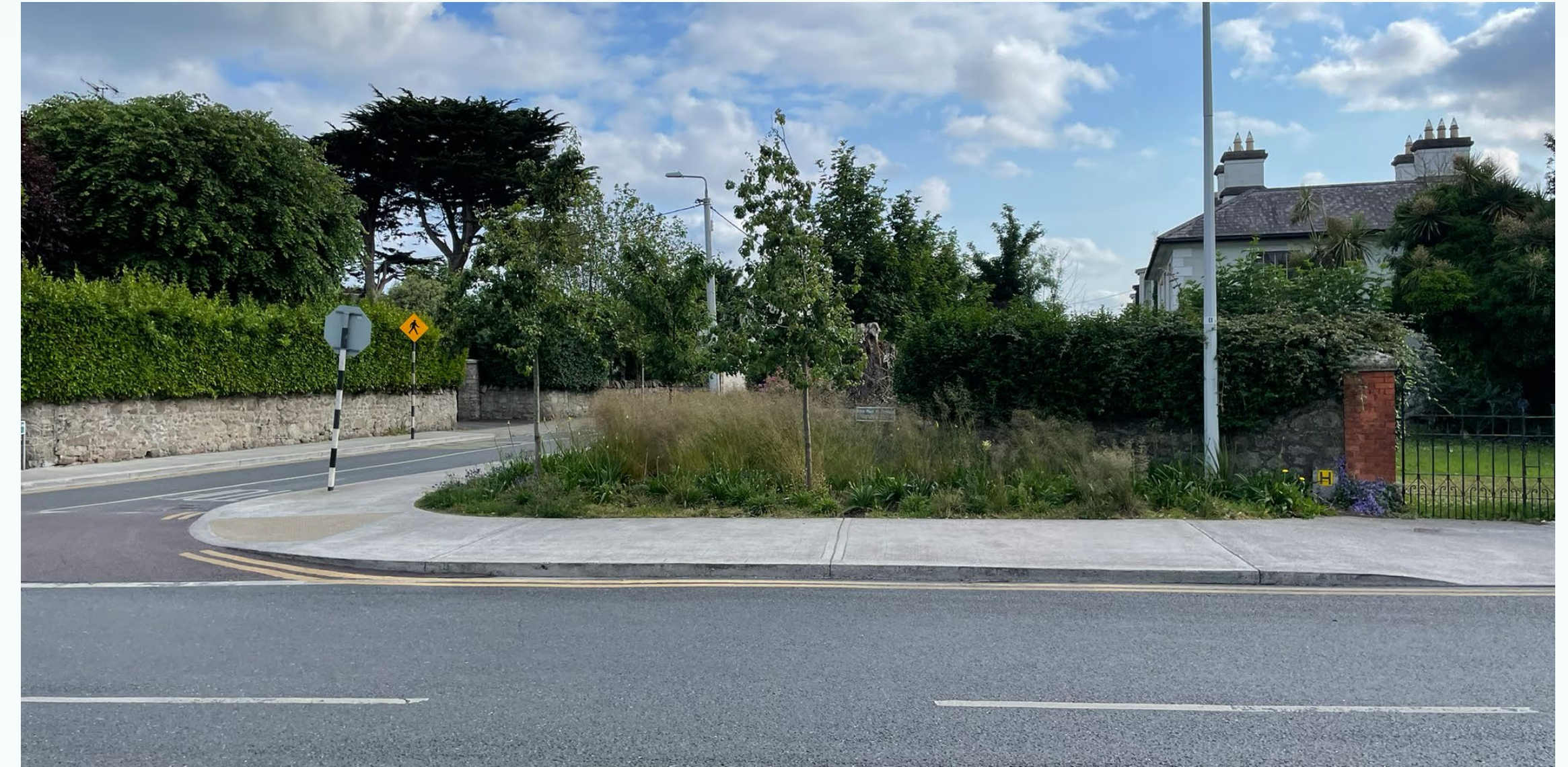
Figure 77: Landscaping area built within space gained from a junction corner radius reduction, Bullock, Co. Dublin Link: © Google Street View 2023
