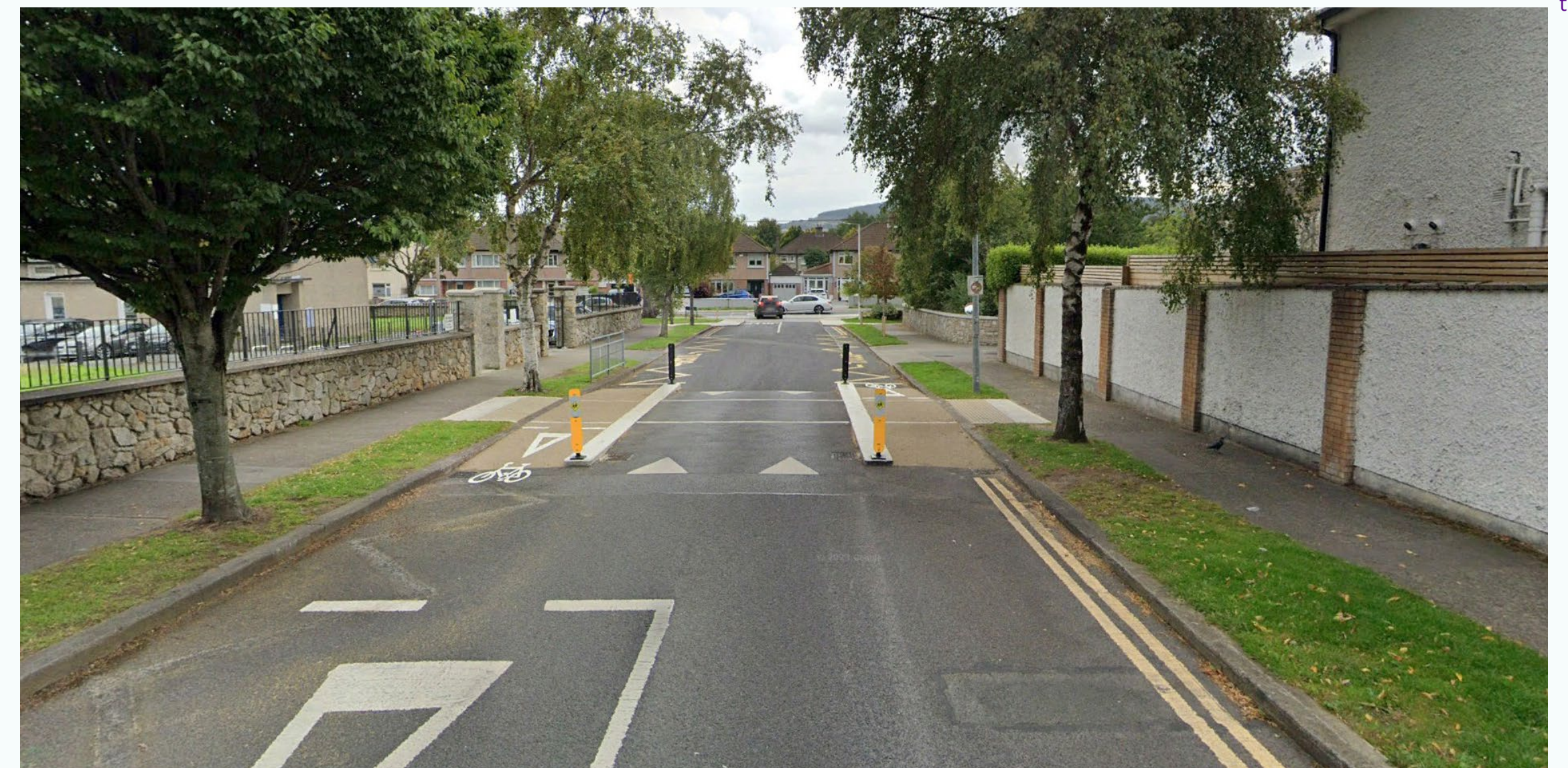
Figure 54: Carriageway Narrowing through a pinch point with a cycle bypass, Dublin Source: © Google Street View 2022
