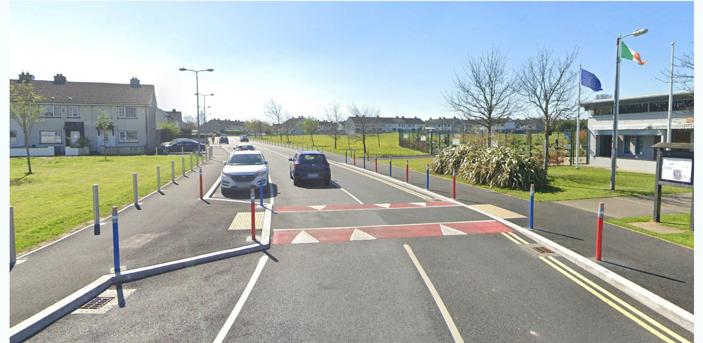
Figure 63: Mid-block raised table with red pavement markings to highlight the ramp, Newbridge, Co. Kildare Source: © Google Street View 2023
