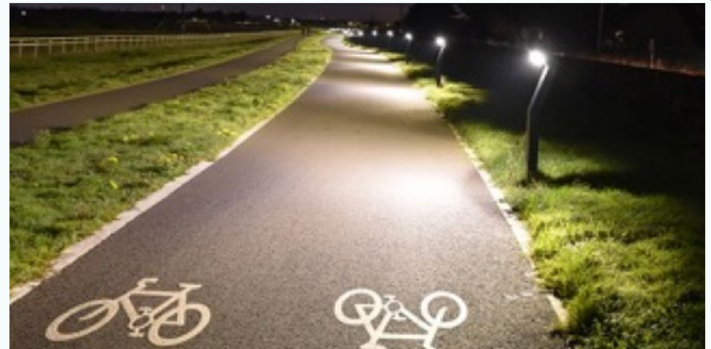
Figure 86: Low level directional lighting along the Portmarnock to Baldoyle Greenway, Dublin
