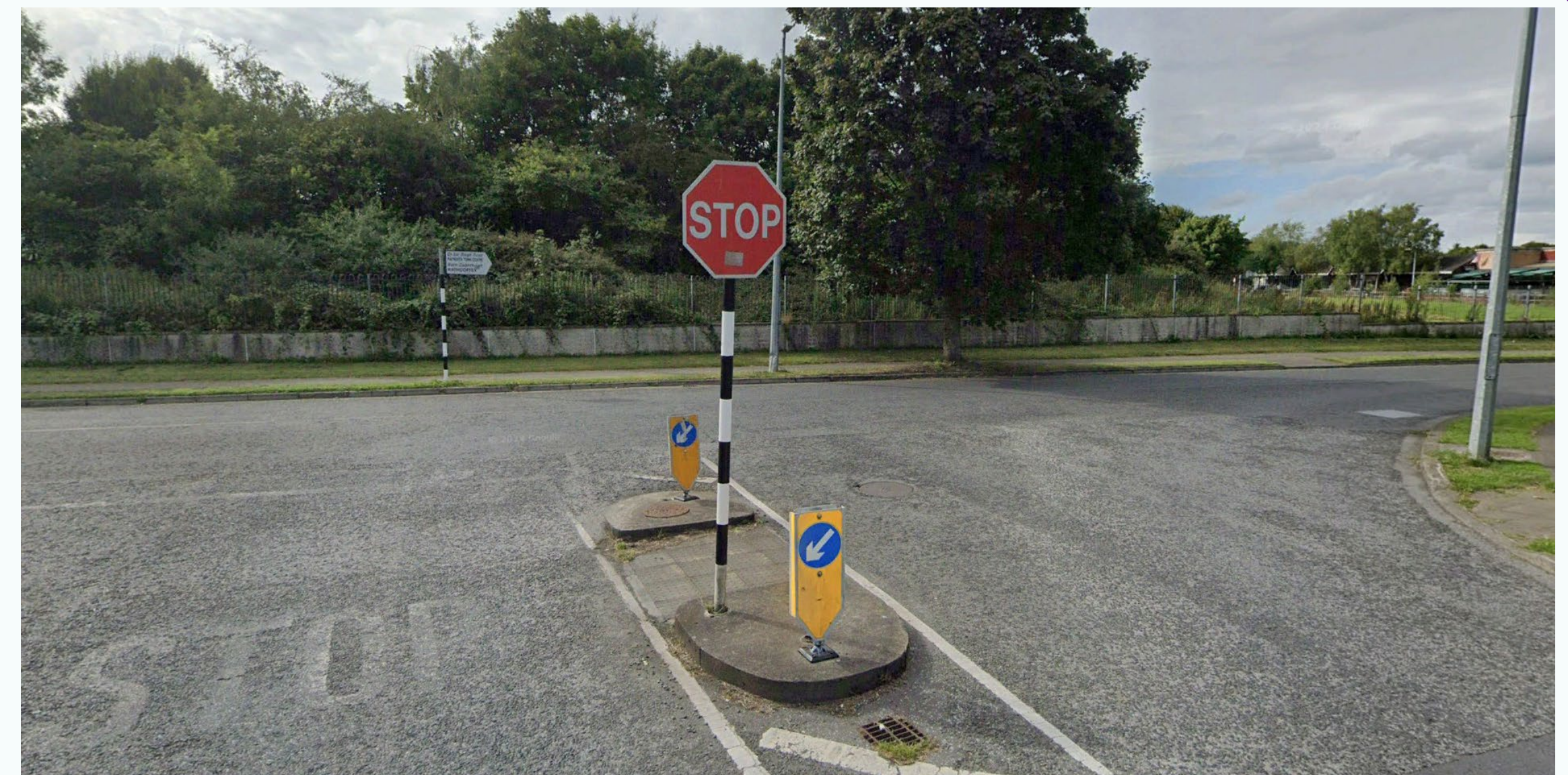
Figure 58: Refuge island at wide junction, Maynooth, Co. Kildare Source: © Google Street View 2024
