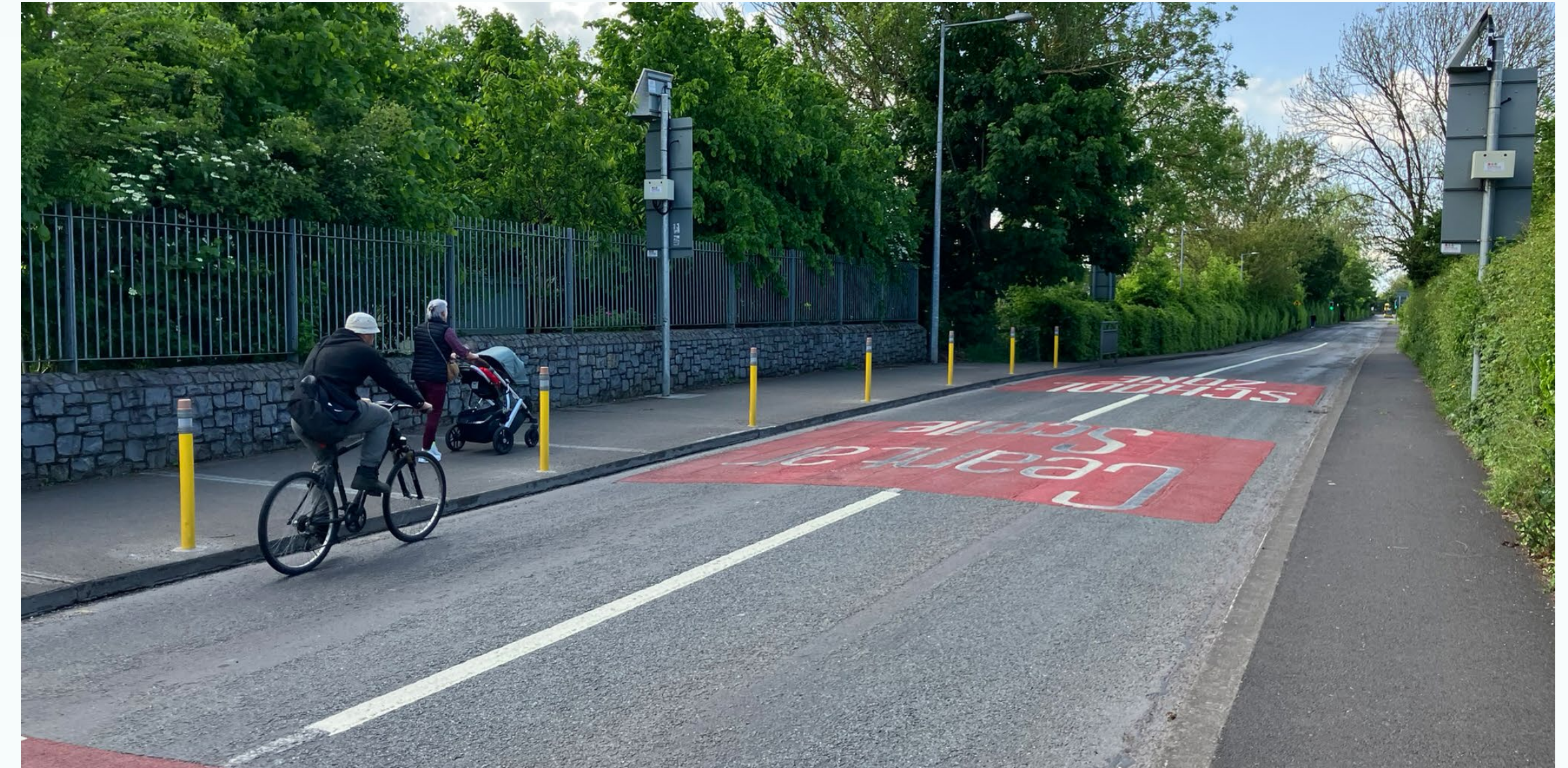
Figure 69: School Zone with decorative bollards, pavement markings and speed humps, Maynooth, Co. Kildare Link: © Google Street View 2024 (image shows the upgrade of existing layout on Google Maps)
