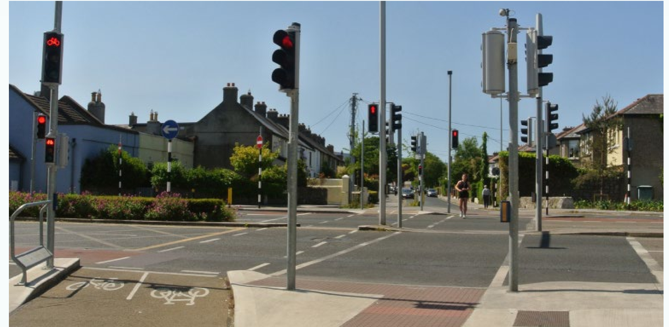
Figure 91: Signalised parallel crossing, Blackrock, Co. Dublin Source: Cycle Design Manual Link: © Google Street View 2022
