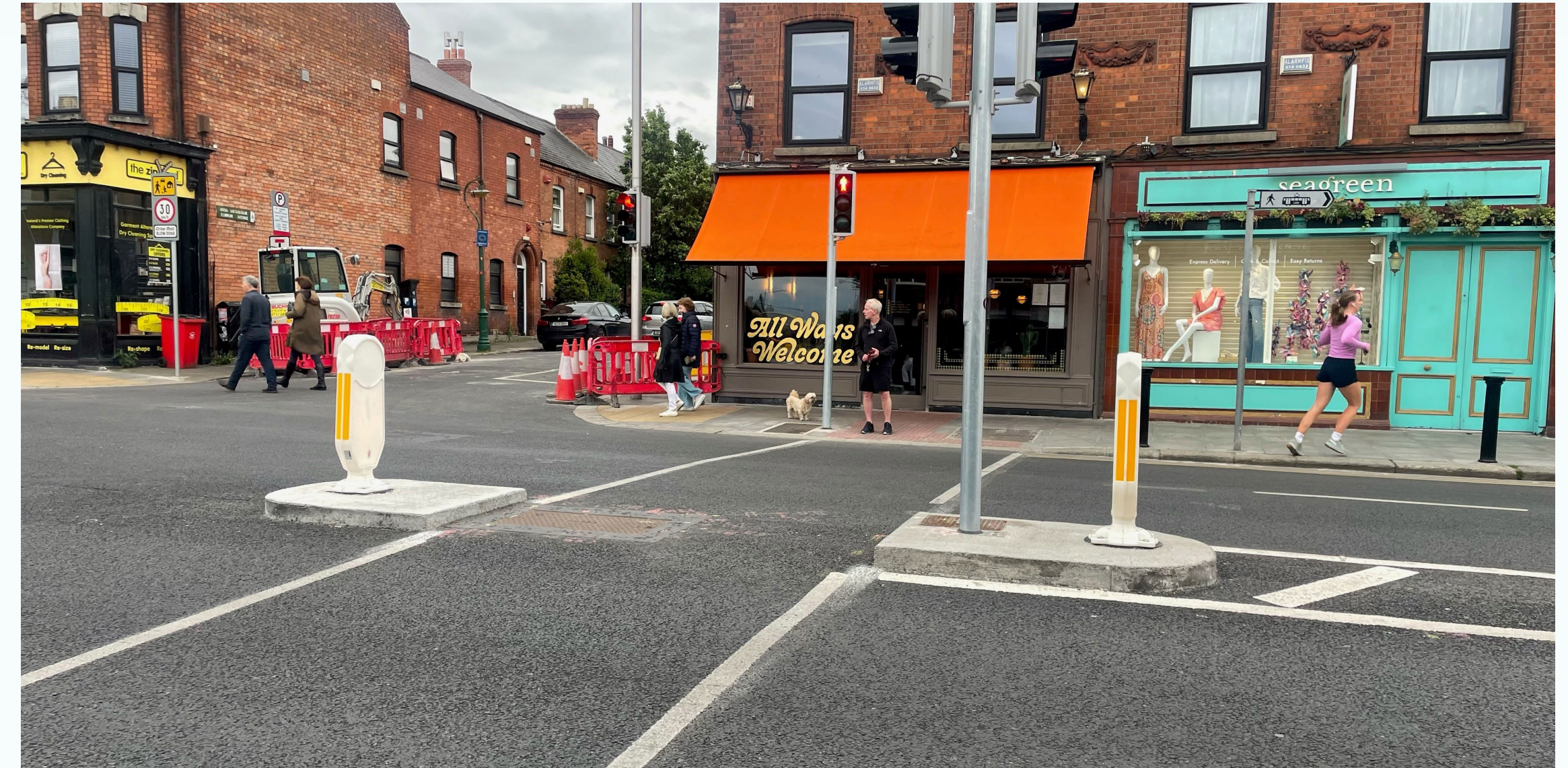
Figure 57: Refuge Island as a signalised pedestrian crossing, Dublin Link: © Google Street View 2022
