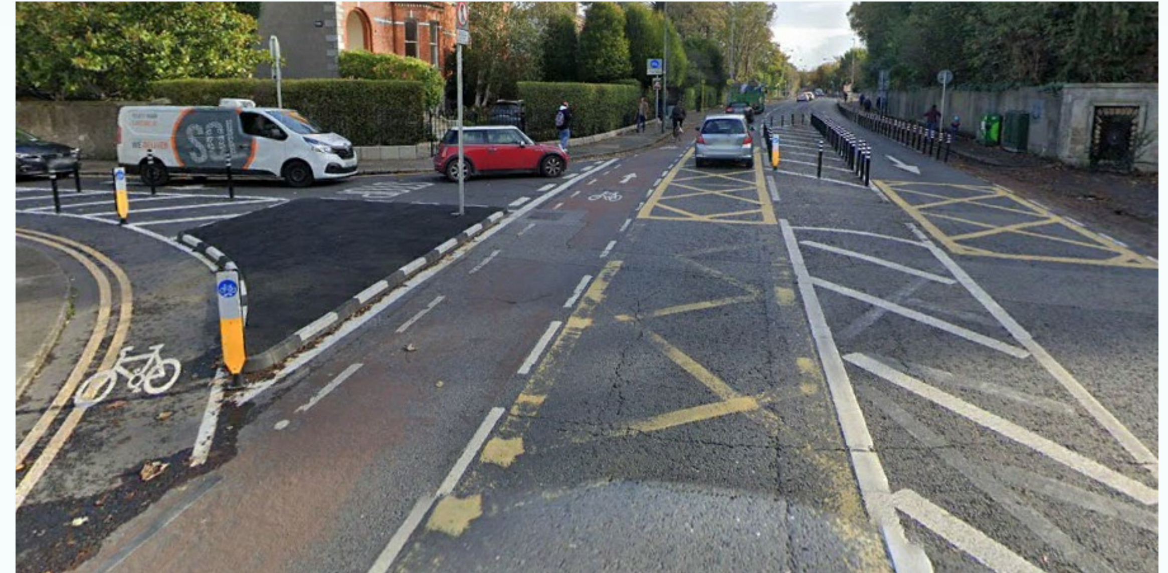
Figure 26: Left Turn Restriction implemented with build-out, cycle bypass for left turning cyclists, Dublin Source: © Google Street View 2022
