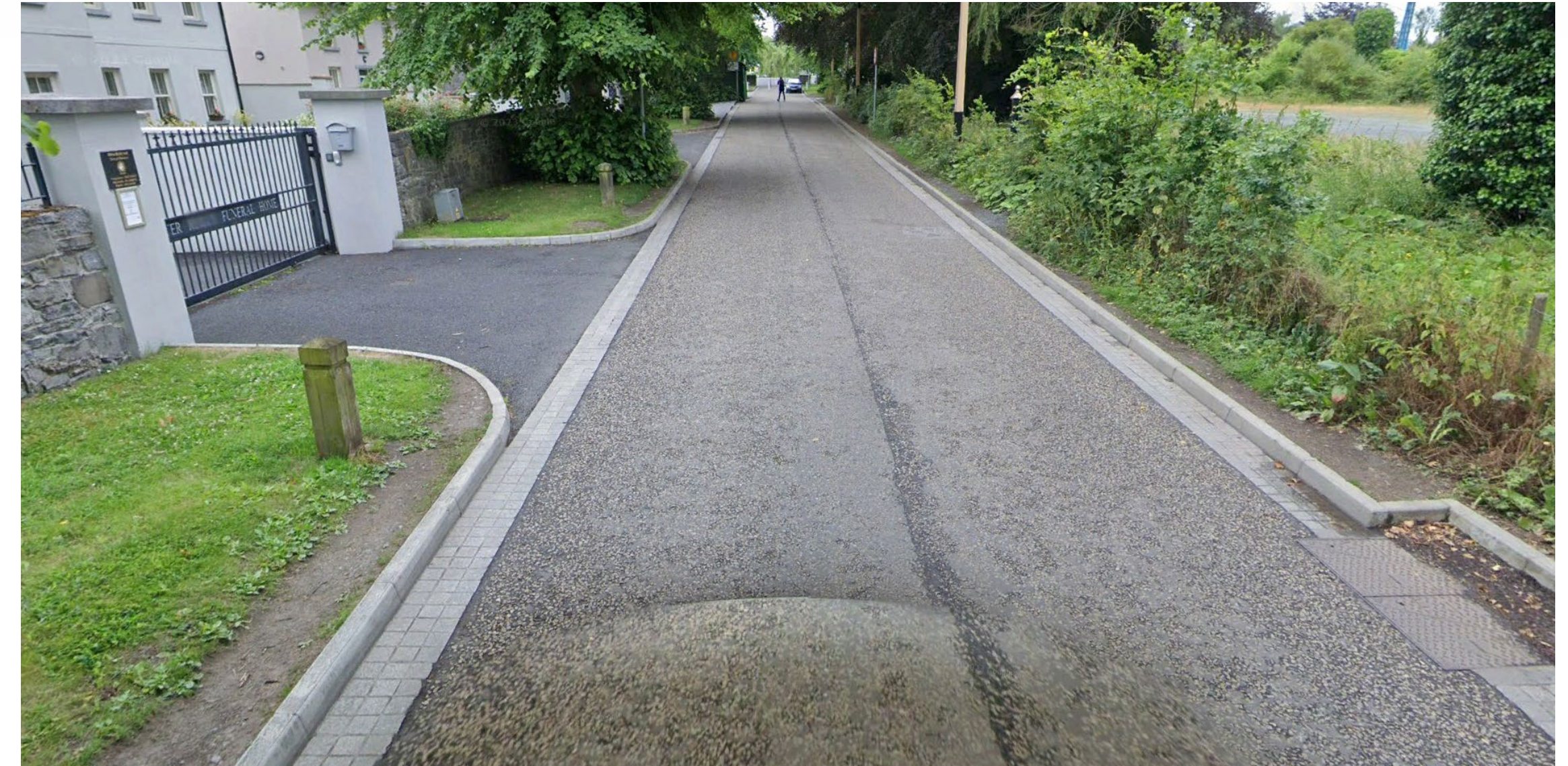
Figure 75: Unit pavers, planting at the edge of the carriageway, and buff coloured pavement act as a form of visual narrowing, Maynooth, Co. Kildare Source: © Google Street View 2023
