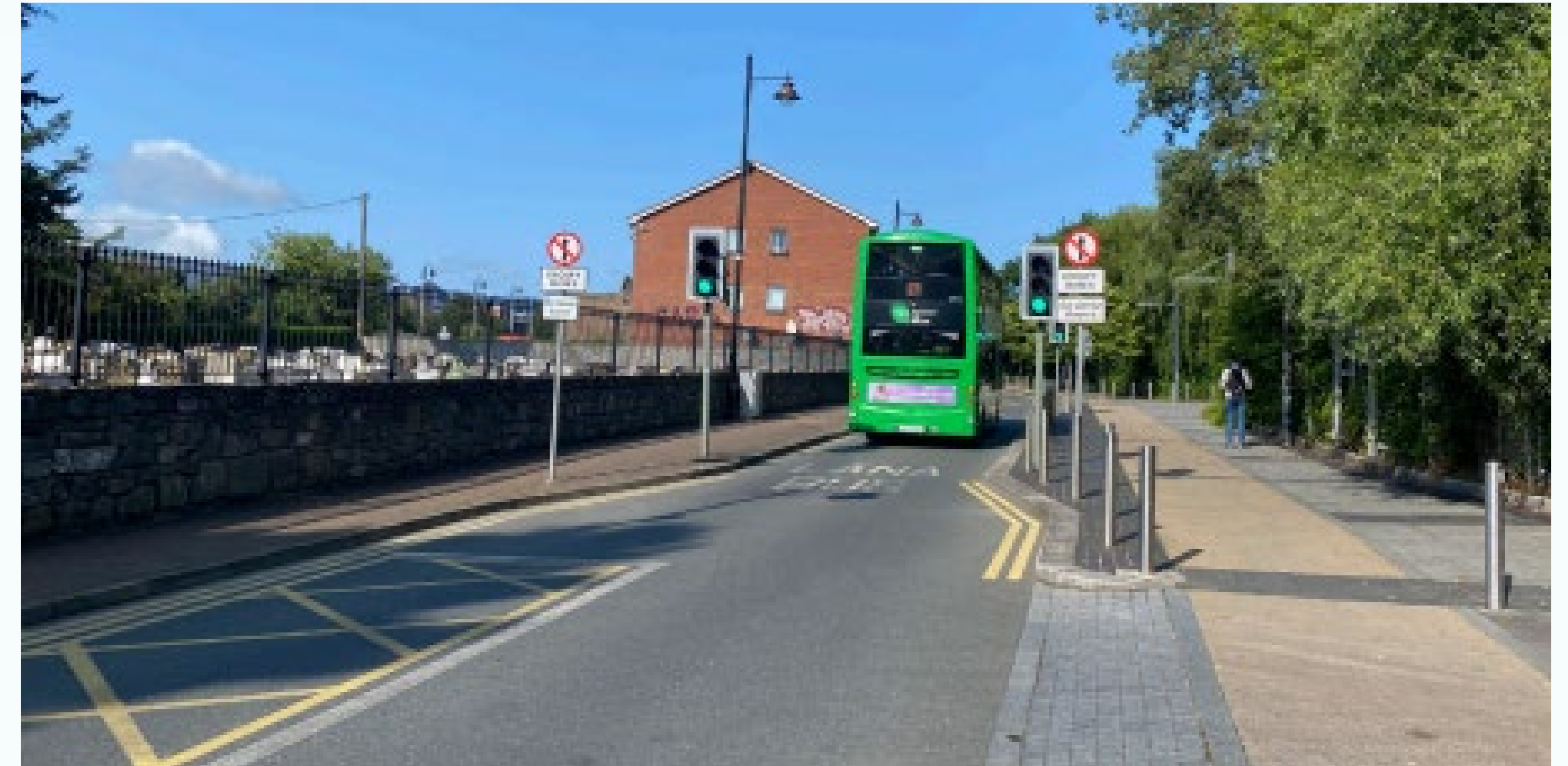
Figure 38: Two-way single lane bus gate on Main Street, Tallaght, Dublin Source: © Google Street View 2022
