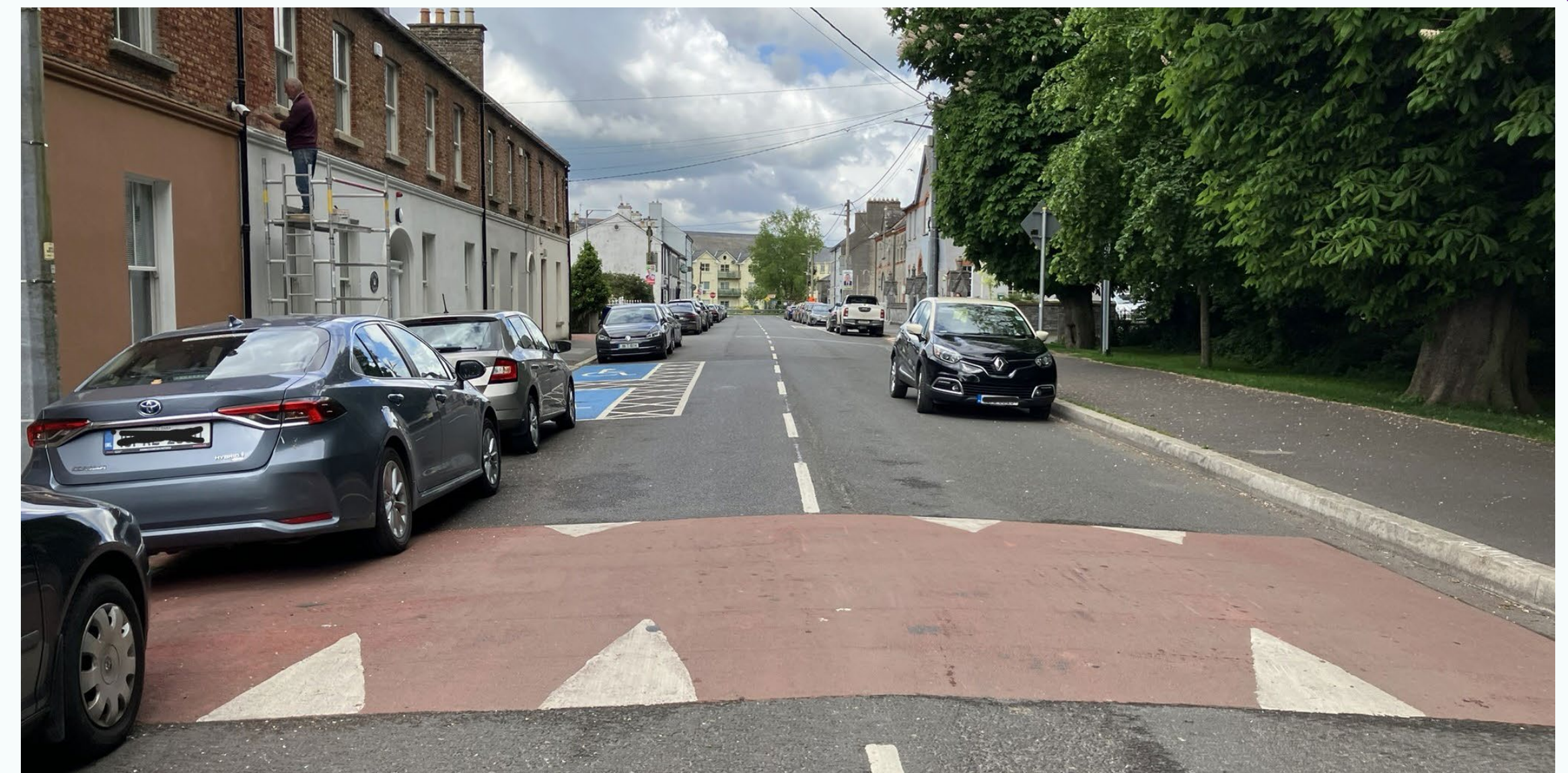
Figure 62: Speed hump in a school zone highlighted with red pavement, Monasterevin, Co. Kildare Link: © Google Street View 2019
