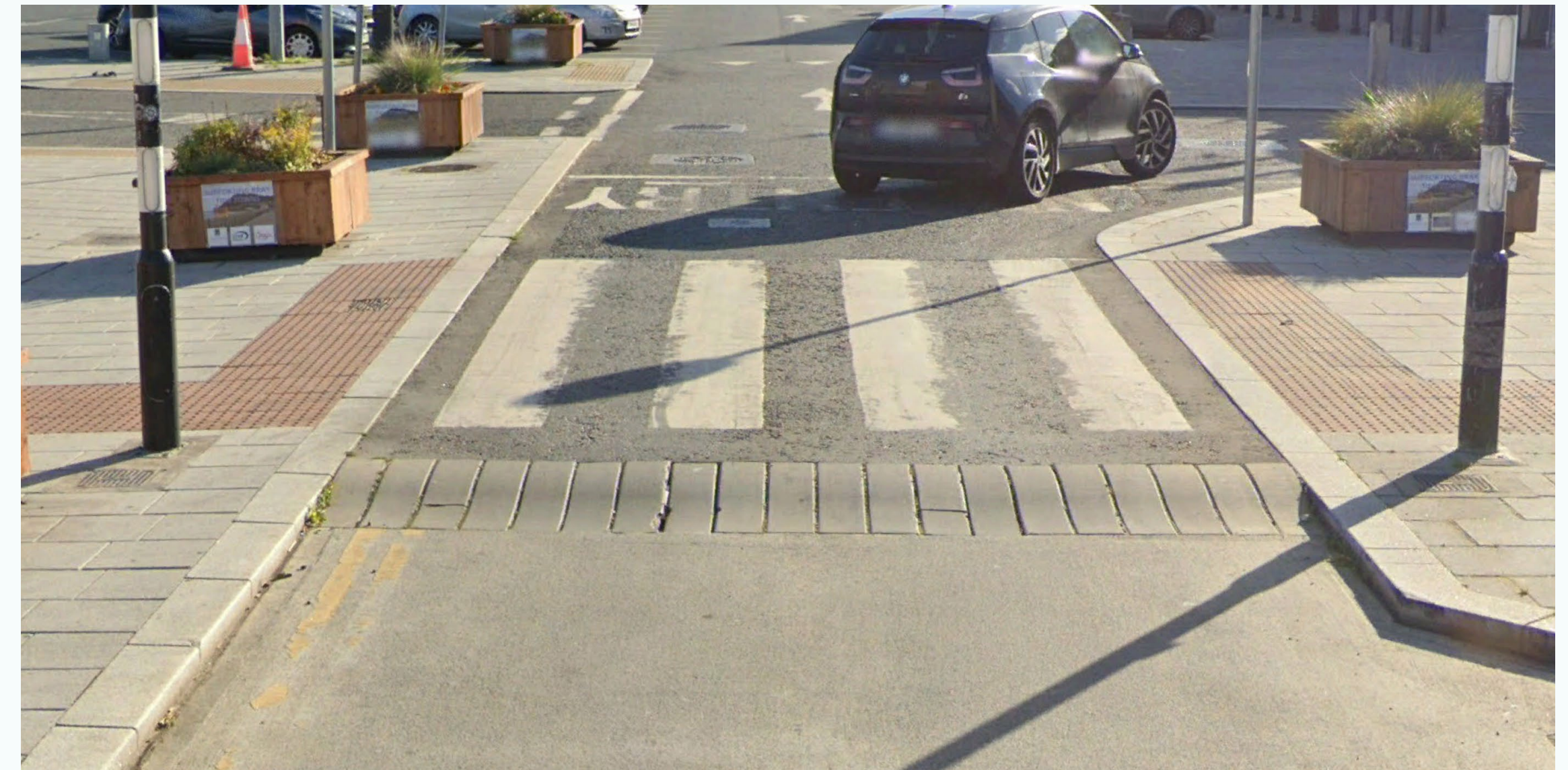
Figure 61: Sinusoidal ramp, Bray, Co. Wicklow Link: © Google Street View 2021
