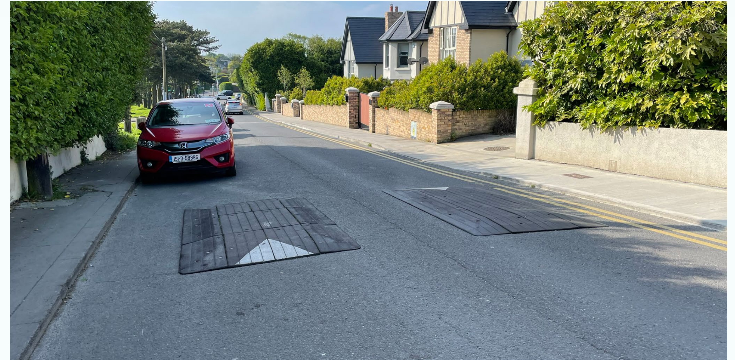
Figure 65: Rubber speed cushions, Howth, Co. Dublin Link: © Google Street View 2023
