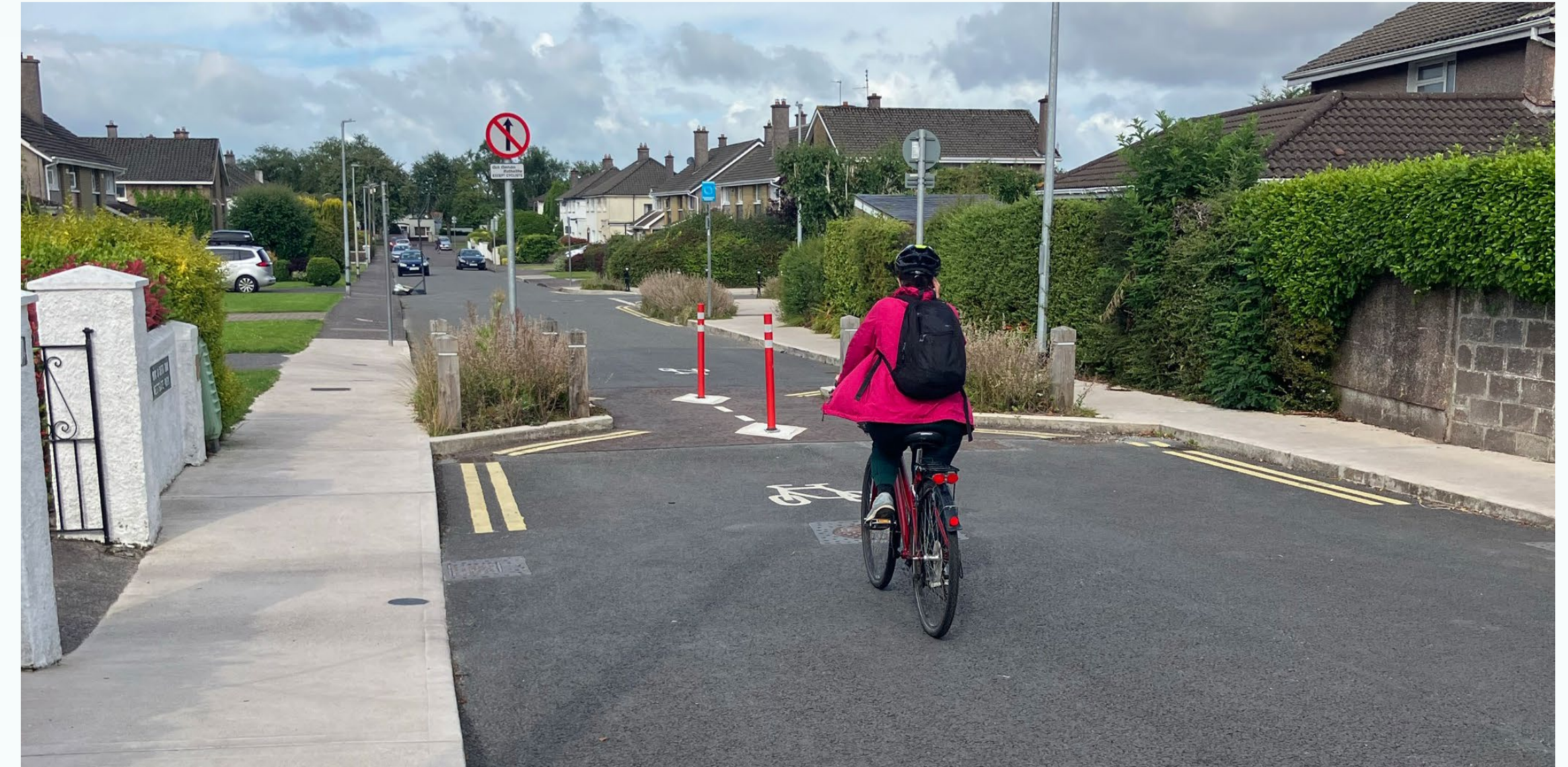
Figure 22: Modal filter with flexible bollards and a build out, Cork Link: © Google Street View 2022 (image shows the upgrade of existing layout on Google Maps)
