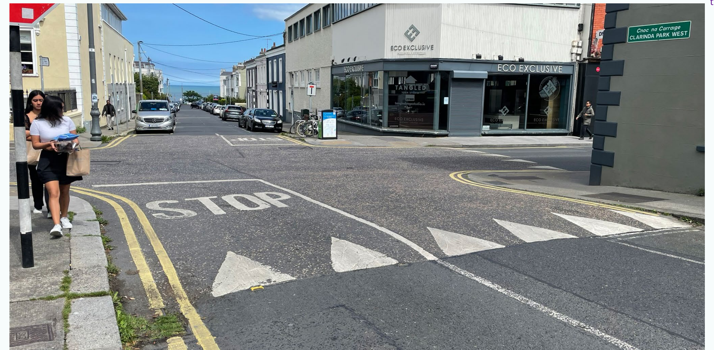
Figure 64: Raised junction, Dún Laoghaire, Co. Dublin Link: © Google Street View 2019
