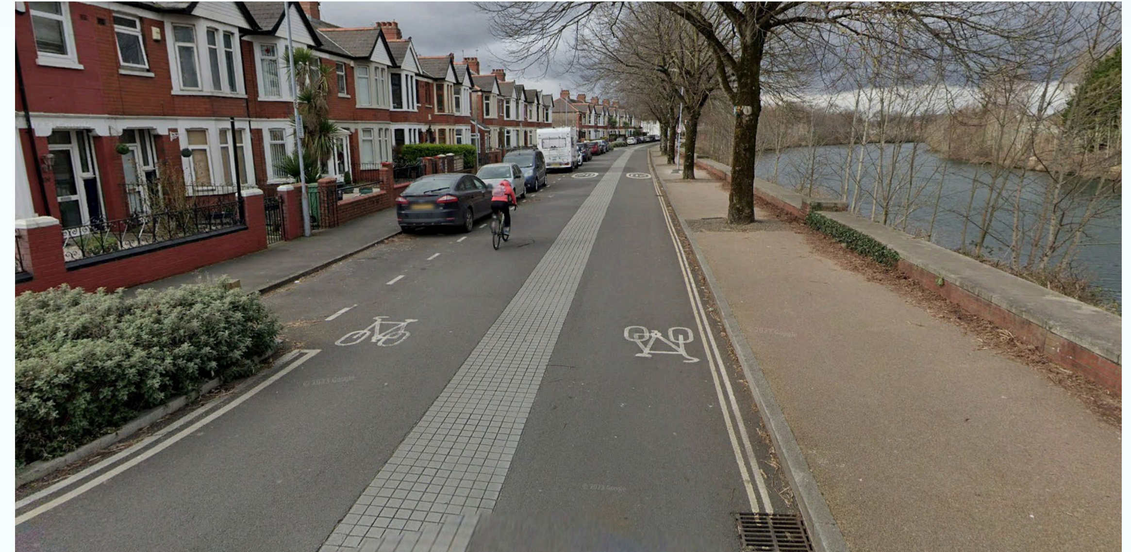
Figure 71: Cycle Street with textured central strip, Cardiff, Wales Source: © Google Street View 2019
