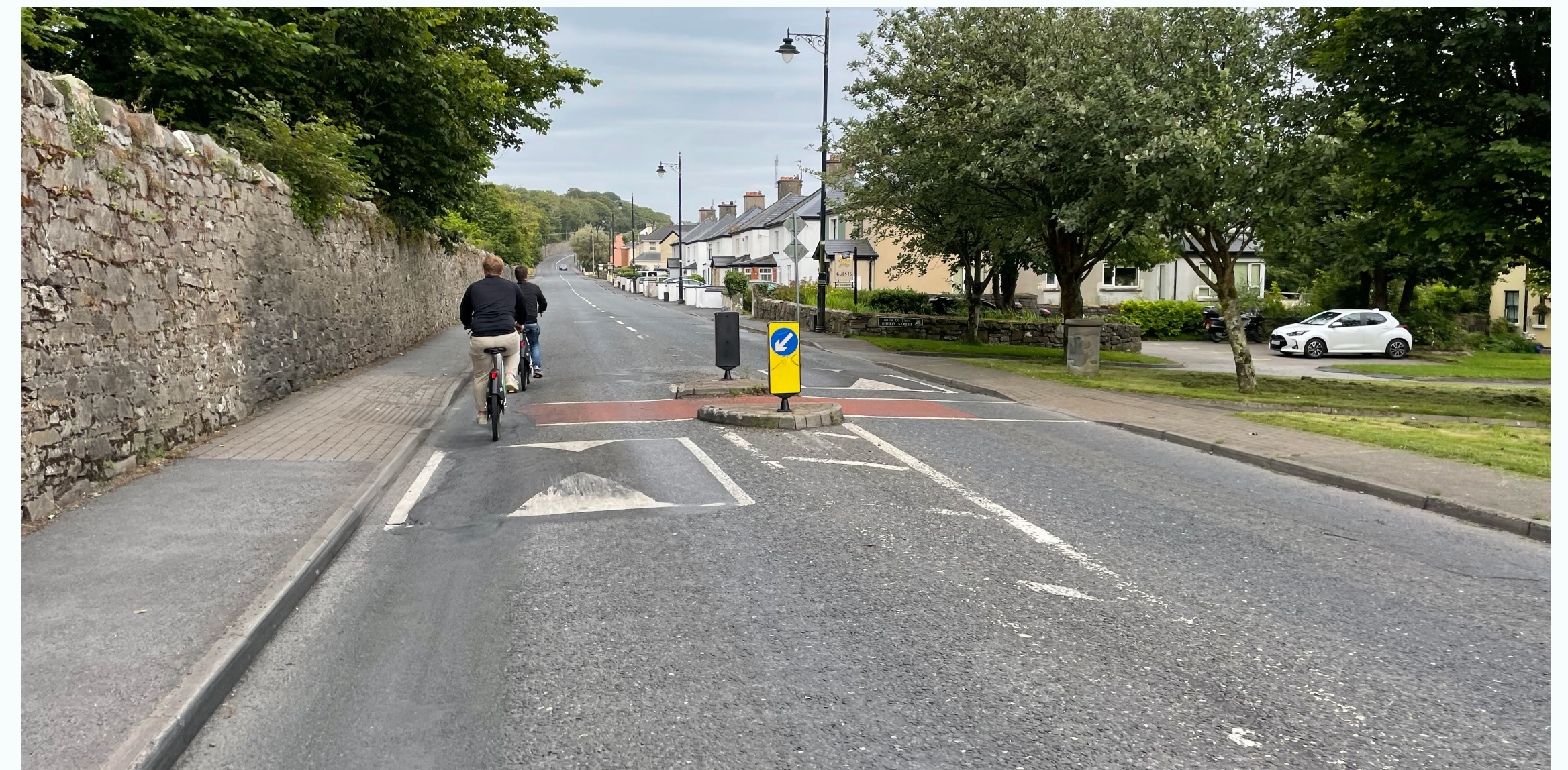
Figure 66: Speed cushions paired with a refuge island, Westport Co. Mayo Link: © Google Street View 2024
