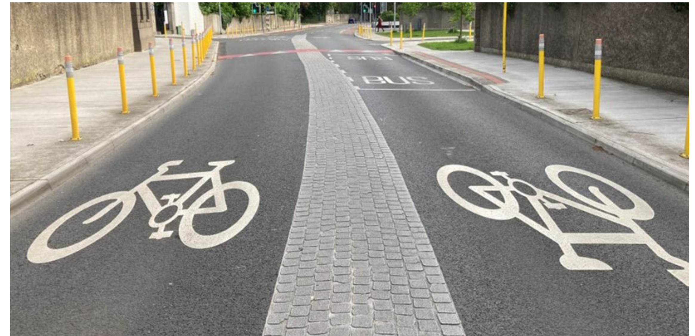
Figure 76: Bollards at the edge of the carriageway and textured central strip provide visual narrowing, Dublin Link: © Google Street View 2022 (image shows the upgrade of existing layout on Google Maps)
