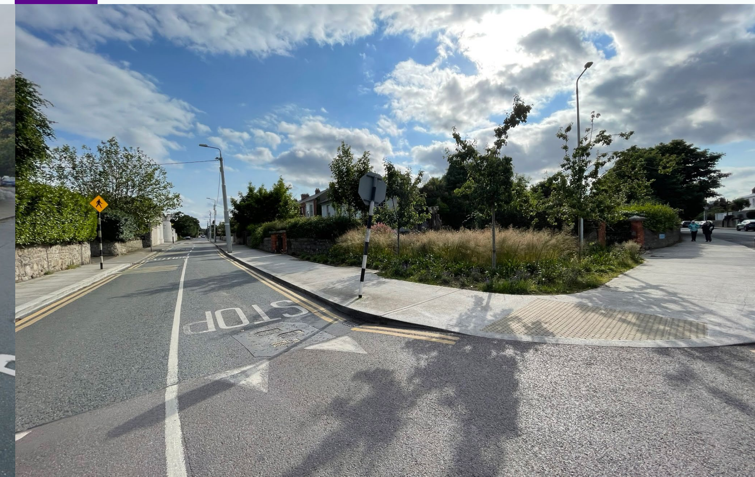
Figure 48: Corner radius reduction through reconstruction provided space for landscaping behind the footpath, Bullock, Co. Dublin Source: © Google Street View 2019 (Before), 2022 (After)
