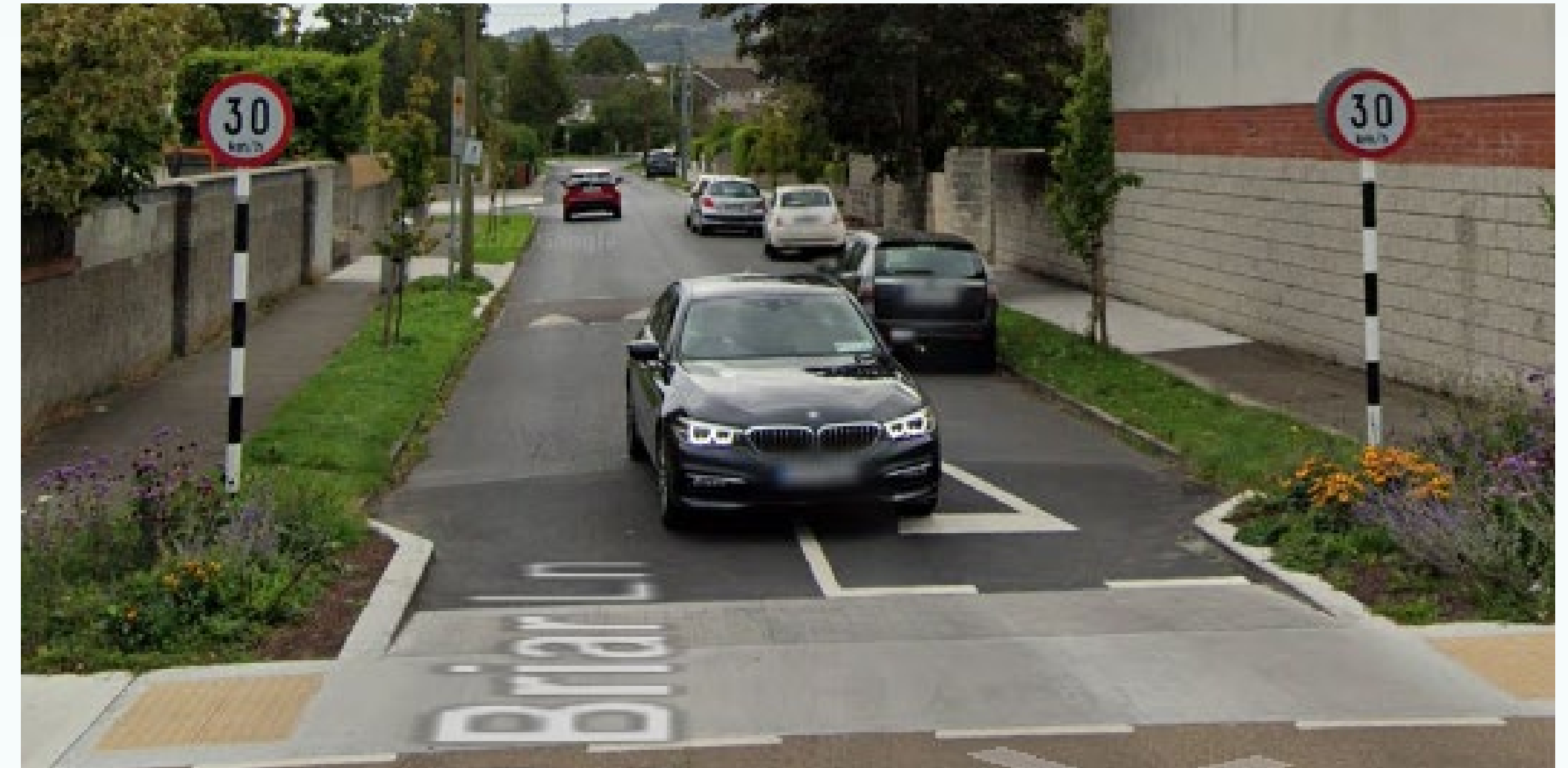
Figure 67: 30km/h speed limit complimented with physical traffic calming measures, Dublin Source: © Google Street View 2022
