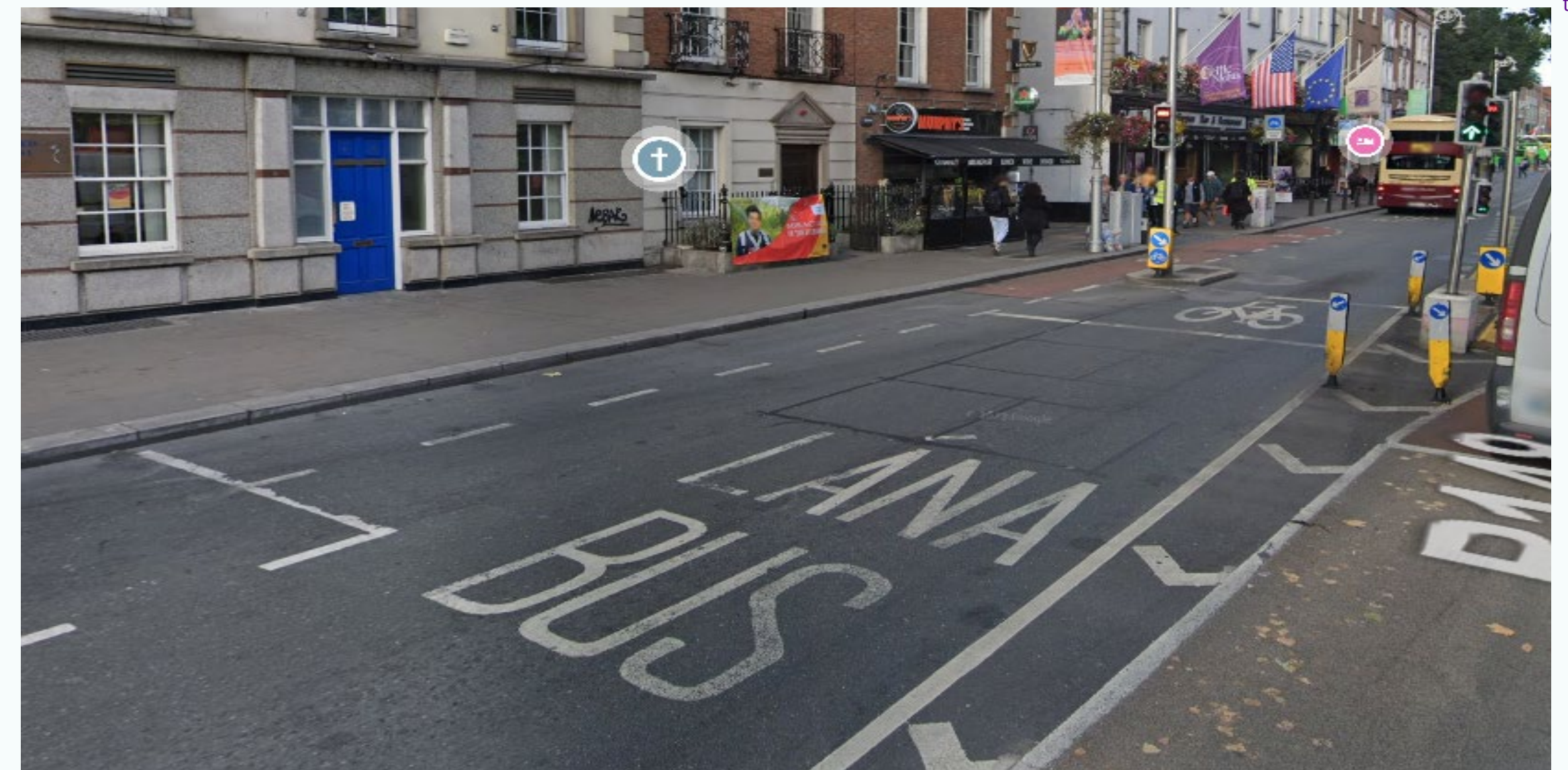
Figure 39: One way bus gate, Dublin Source: © Google Street View 2022
