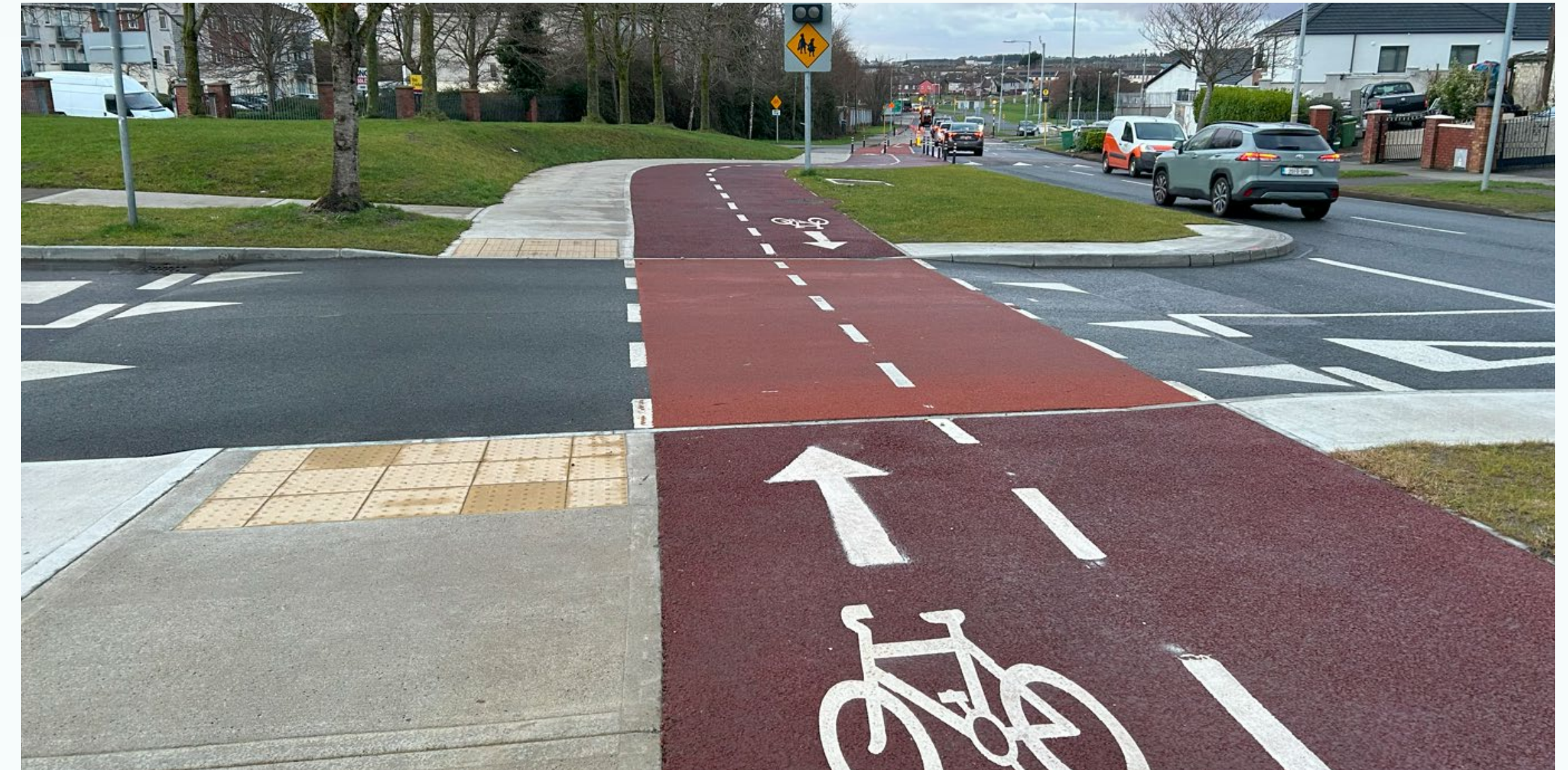
Figure 51: Raised crossing constructed with unit pavers, Dublin Link: © Google Street View 2024
