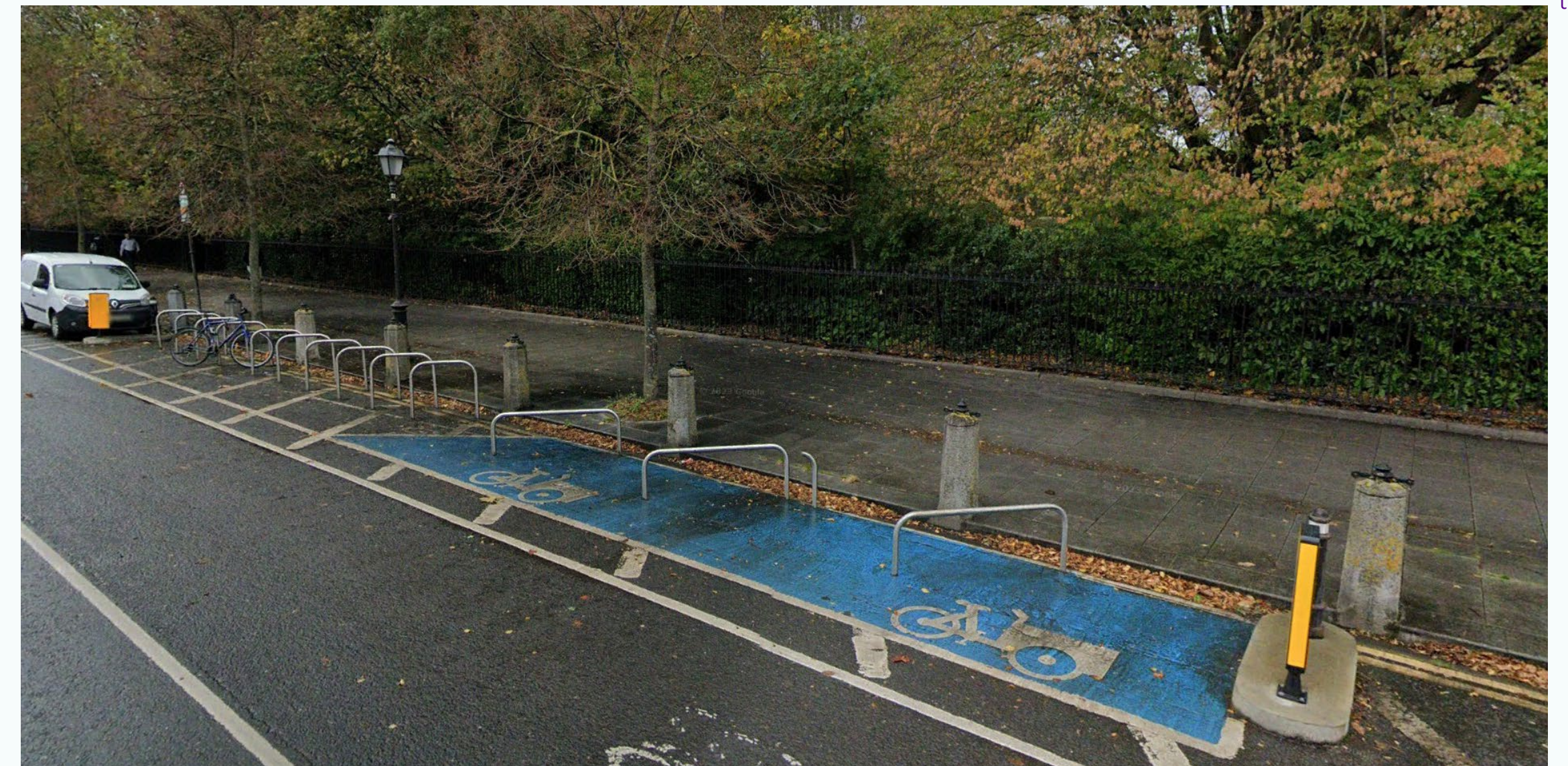
Figure 94: Short stay cycle parking for standard and large cycles within the carriageway, St Stephens Green, Dublin Source: © Google Street View 2022
