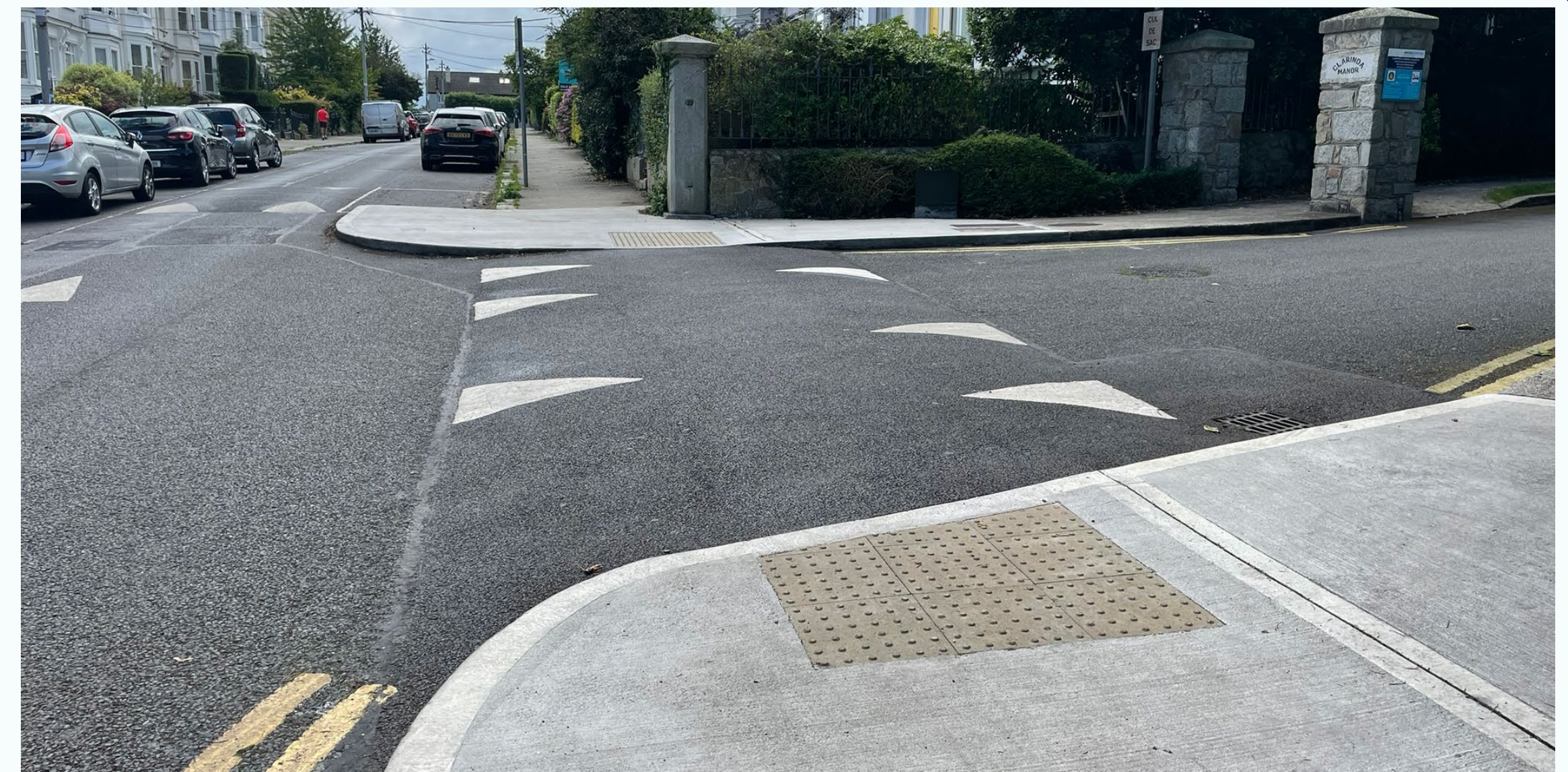
Figure 52: Asphalt raised crossing, Dún Laoghaire, Co. Dublin Link: © Google Street View 2019 (image shows raised crossing not visible on Google Maps)
