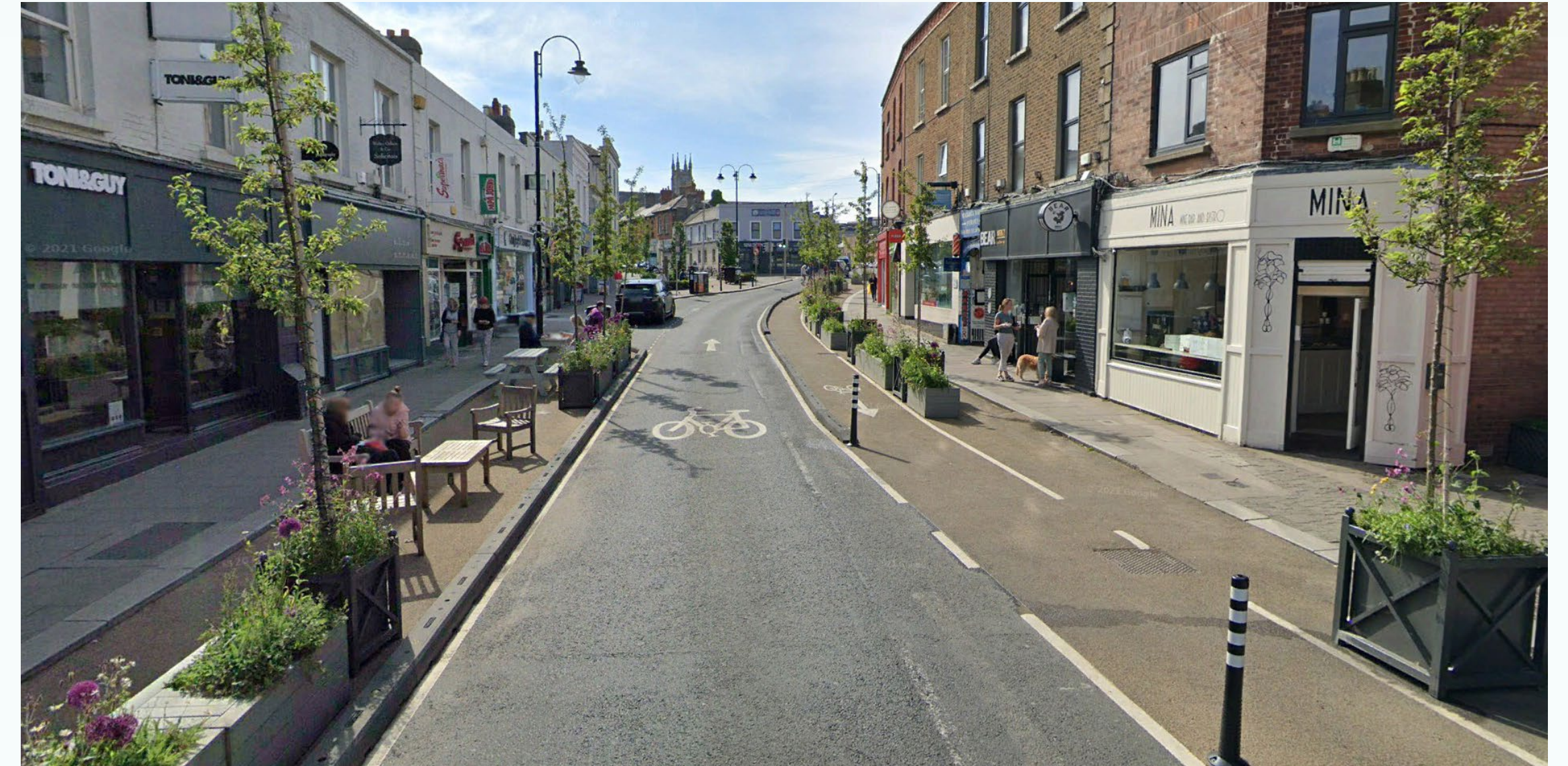
Figure 53: Carriageway narrowed by build-outs and a protected contraflow cycle lane, Blackrock, Co. Dublin Source: © Google Street View 2021
