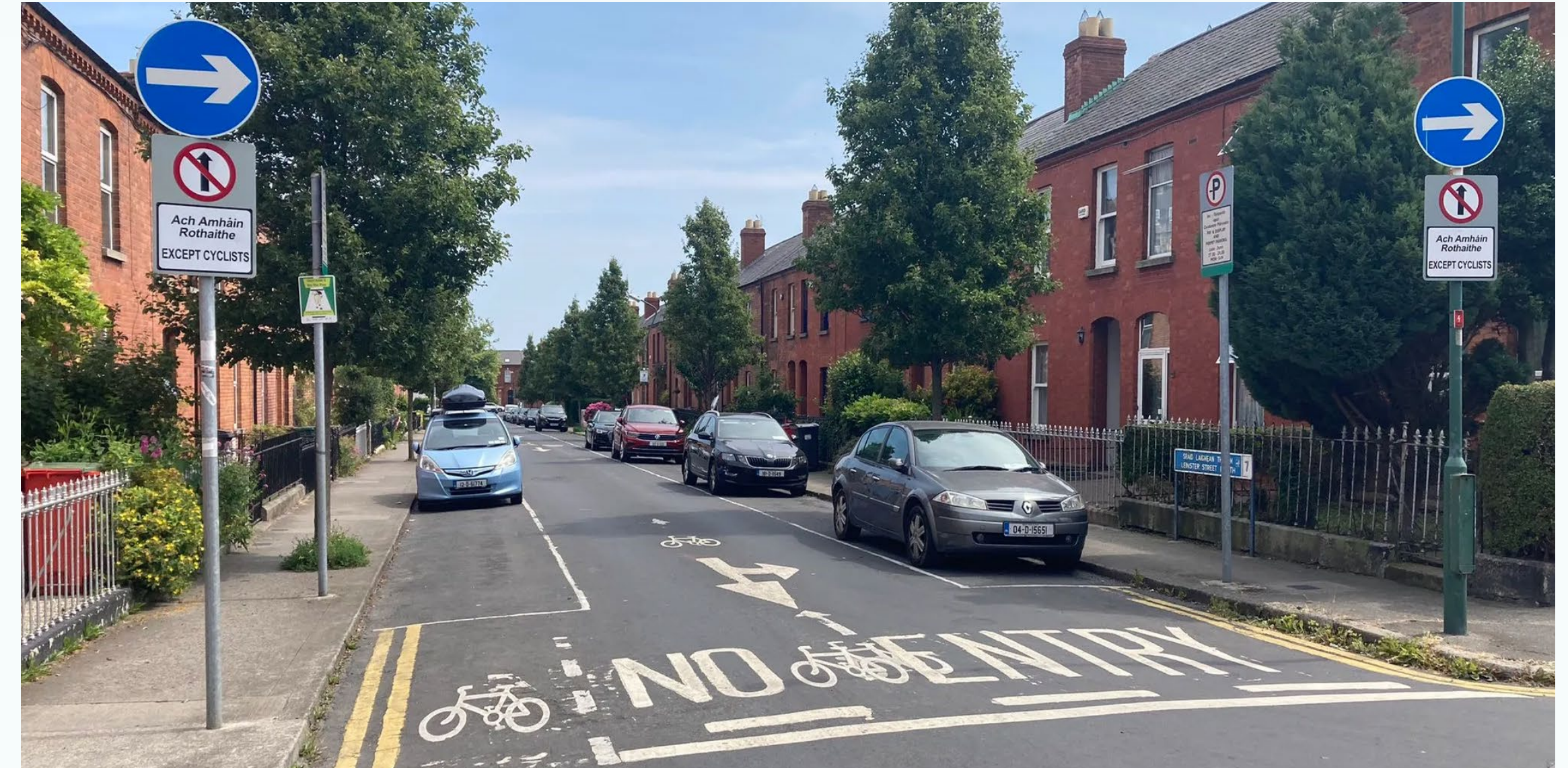
Figure 30: One way street marked by "No-Entry" signs with contraflow cycling permitted, Dublin Source: © Google Street View 2023
