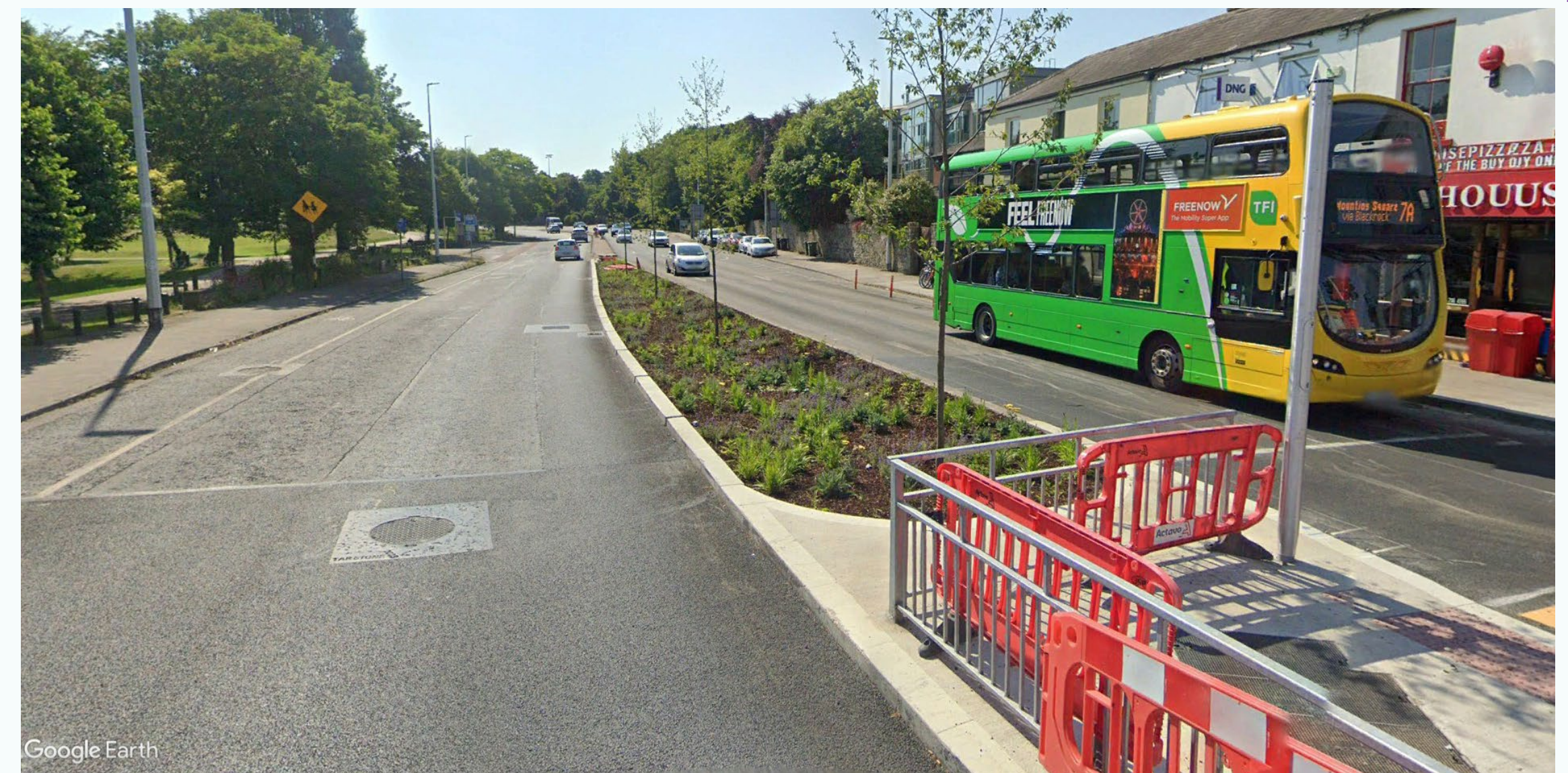
Figure 78: SuDS incorporated into a median, Booterstown, Co. Dublin Link: © Google Street View 2023
